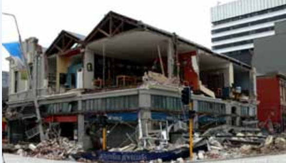
Figure 3.3: Out-of-plane wall failures in longitudinal and transverse directions.
