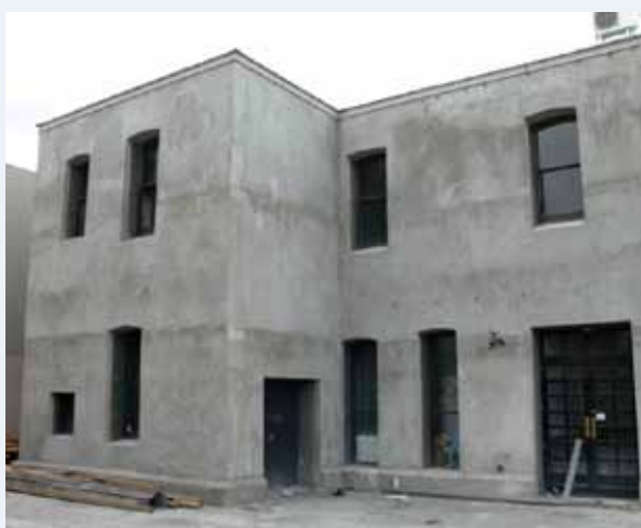
Figure 3.12: Shotcrete applied to a former URM building.
