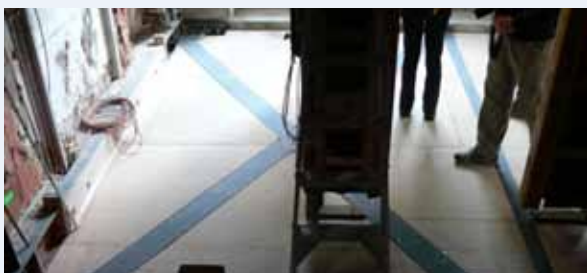
Figure 3.10: Steel strapping for floor stiffening.
