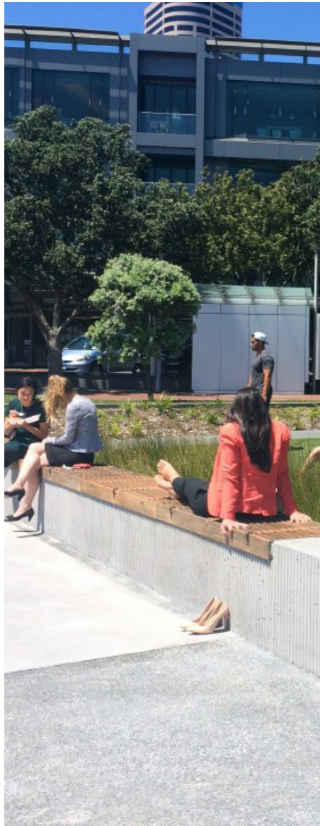
CONCRETE SEATING WALL WITH TIMBER INSET
