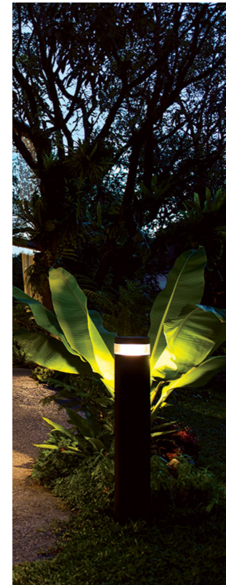
ACCESSWAY AND BOARDWALK EDGE LIGHTING
