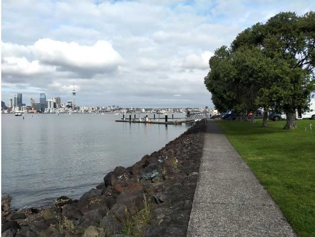
Figure 1 – Looking south to ferry terminal from the boat ramp
