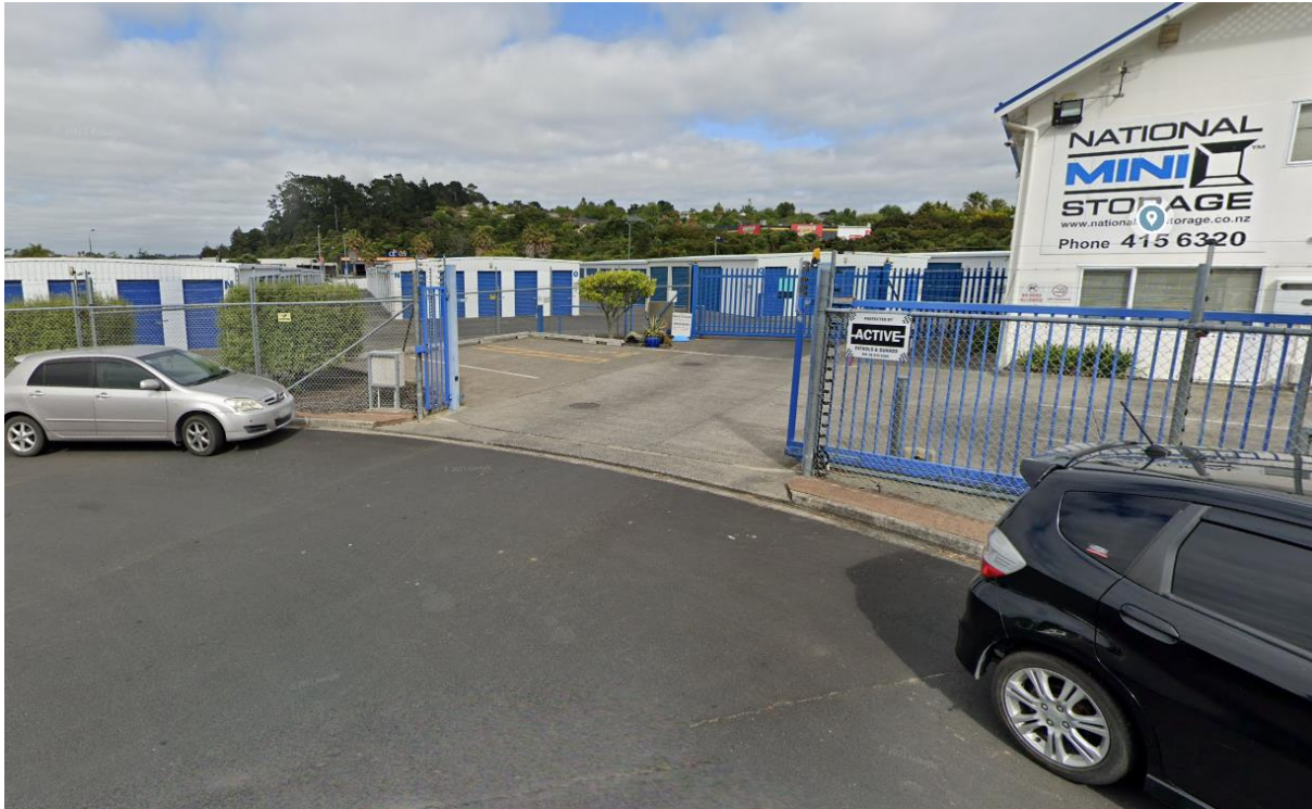
FIGURE 3: NATIONAL MINI STORAGE ALBANY 1 (6 MIRO PLACE, ALBANY, AUCKLAND 0632)
