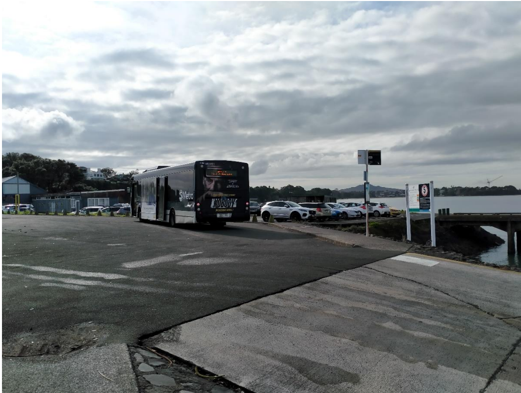
Figure 3 - Looking northeast to bus stop with boat ramp in foreground.
