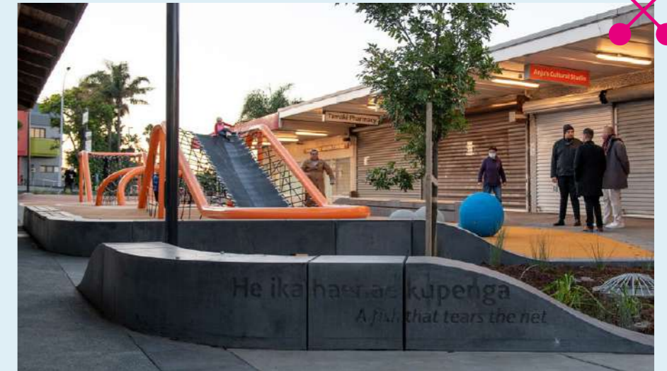
▲ The new space is based on the cultural narrative of the eight-tailed taniwha Moko Ika Hiku Waru, which has been woven into the playground’s design, providing a cultural anchor for the space. The narrative was gifted by Ngāti Pāoa Iwi Trust, along with four whakataukī (proverbs) that have been inscribed in the low concrete walls that run through the court.
