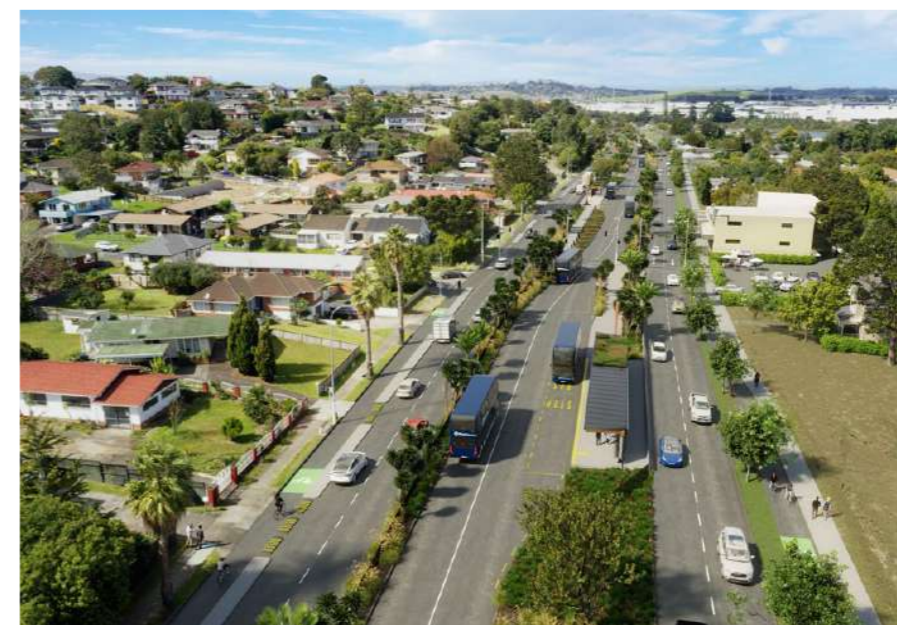
▲ Artist impression of the completed Eastern Busway on Tī Rākau Drive and showing Edgewater Station
