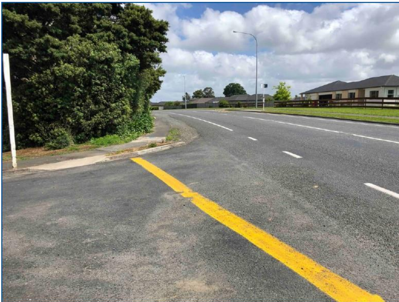
Figure 2: Gatland Road intersection with Great South Road, looking south
