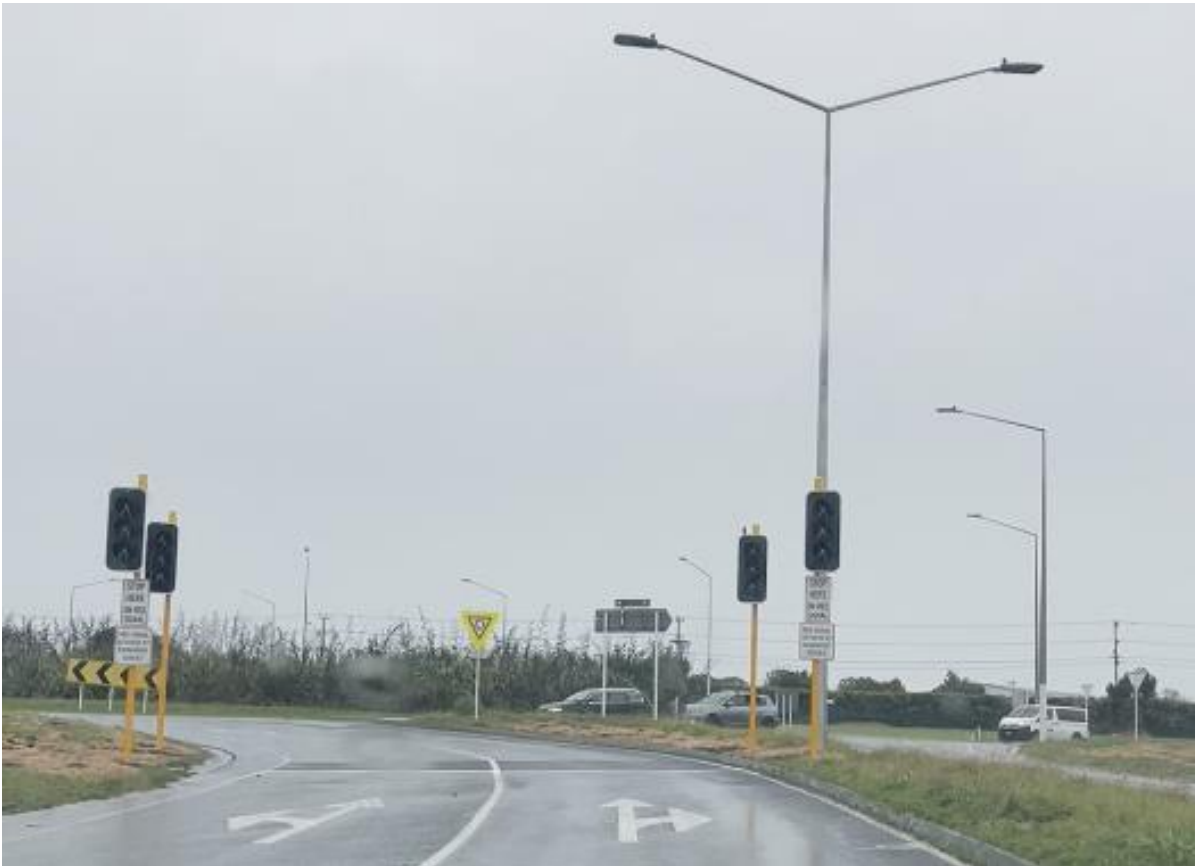
Figure 2: Meter signals installed on the Brigham Creek Road approach to the SH16 Brigham Creek Roundabout
