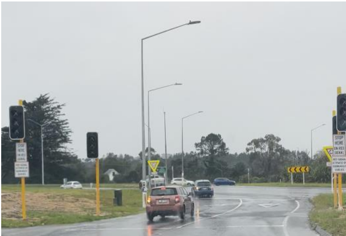
Figure 1: Meter signals installed on the Fred Taylor Drive approach to the SH16 Brigham Creek Roundabout
