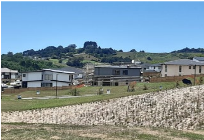
View down the valley showing dwellings in sub-precinct H with 3m side yards [6m gap between dwellings]
