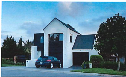
Street elevation incorporating garage doors discretely and presenting a strong formal aspect to the street.
