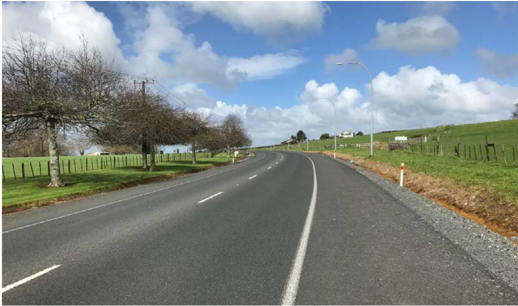
Photograph 2: Southern direction along Buckland Road (northern end)
