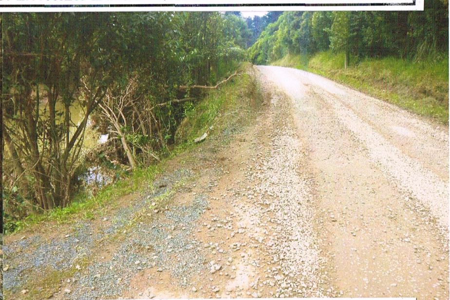
Gravel Road opposite entrance to Quarry
