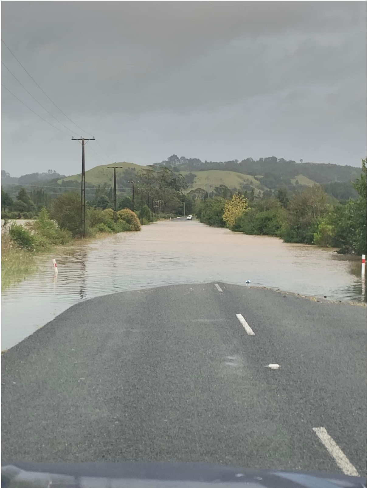
(above: Tourist Road, Clevedon, February 2023 Floods)
