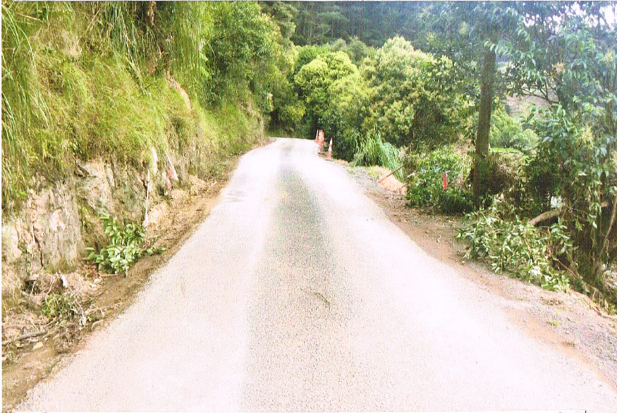
Single Lane Road to Quarry w slip into River
