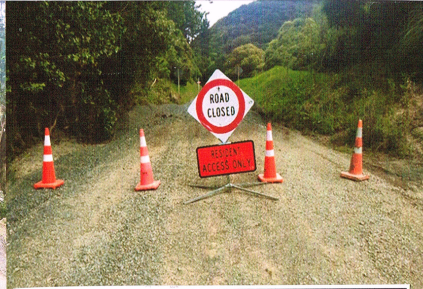
Road 30 metres past the quarry. Out of Service.
