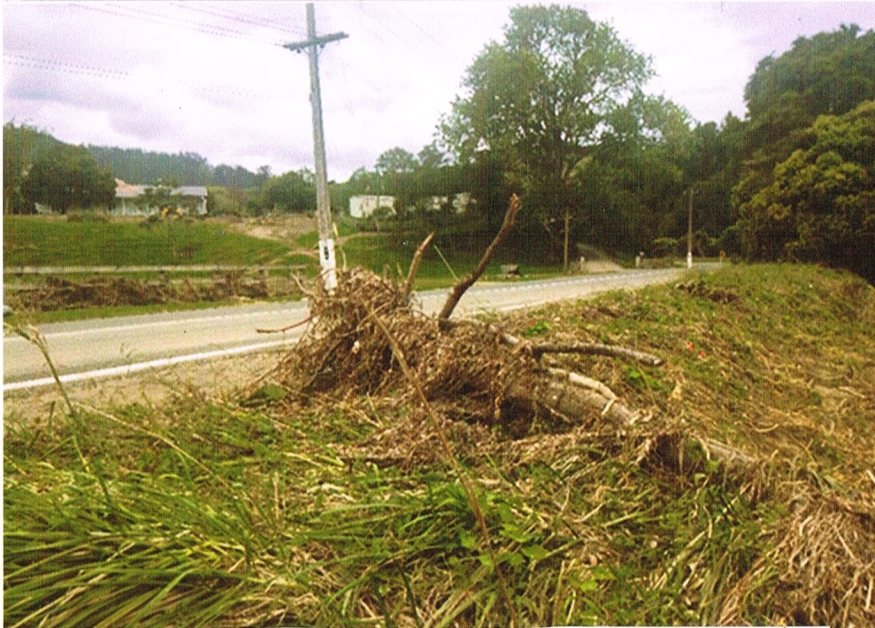
When River floods it covers the road to the Quarry
