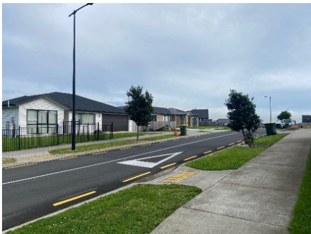
Figure 8: : Typical development within Glenbrook 3 Precinct
