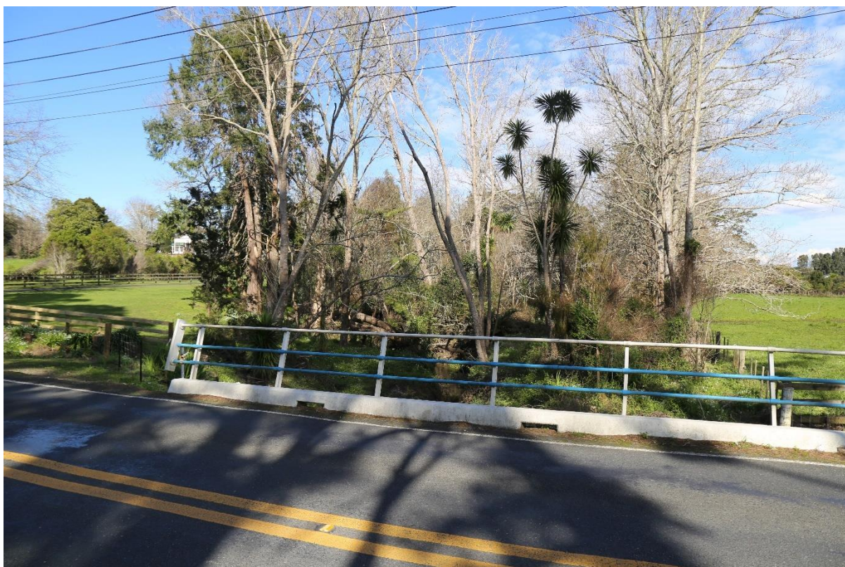
Figure 10-4: Existing vegetation to the south of the existing Access Road bridge.
