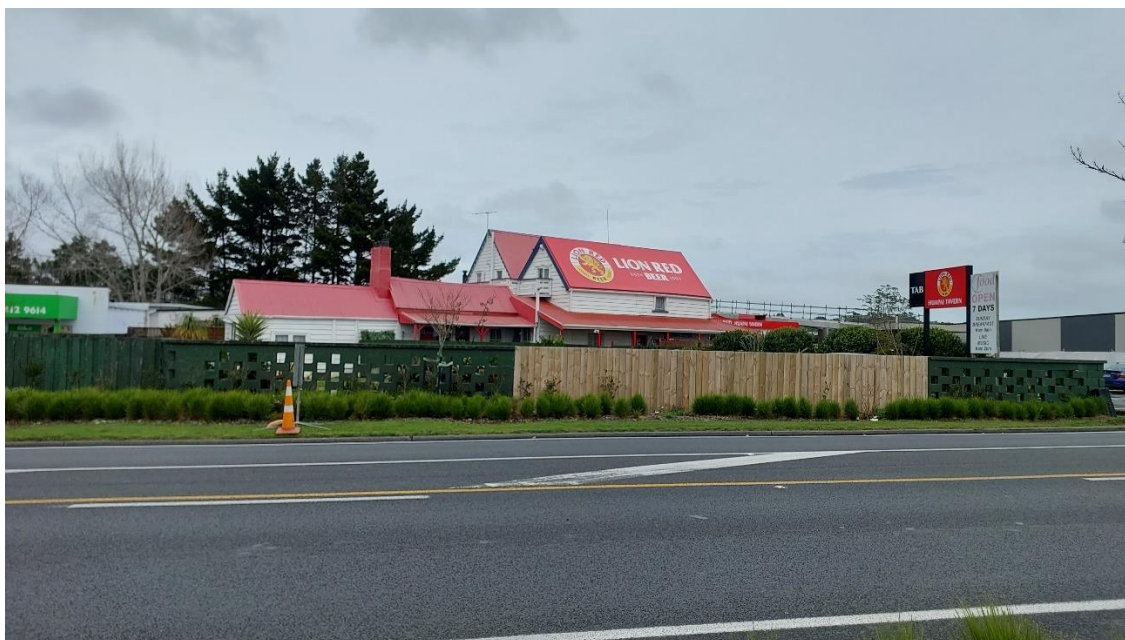
Figure 4-2: Extent of Place for Huapai Tavern extends spatially into the road reserve and may be impacted by construction activities of NoR S2
