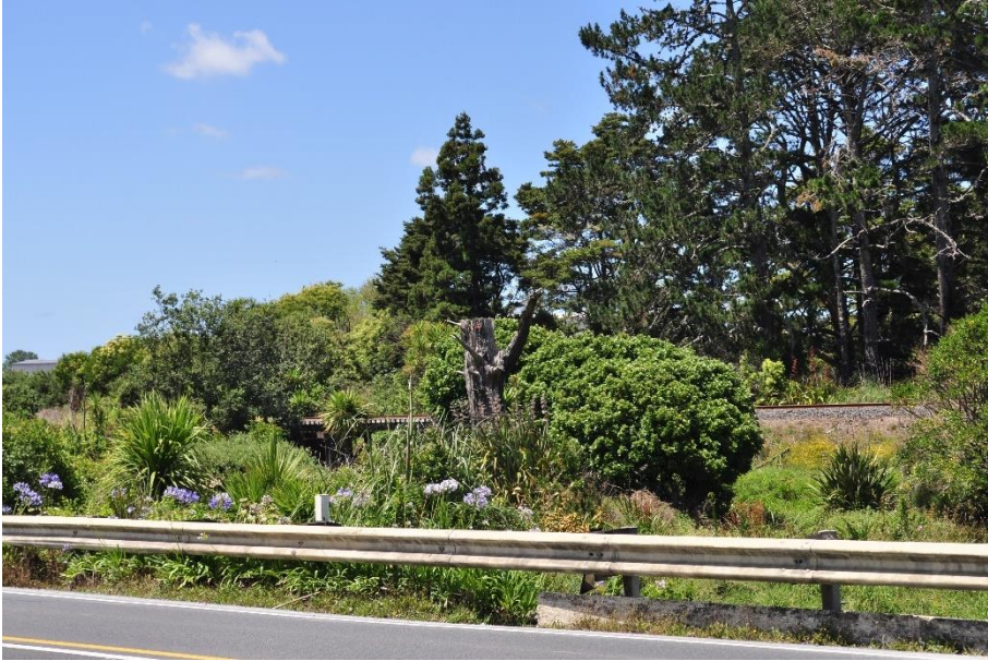
Figure 9-12: Railway bridge over the Turakiawatea stream.
