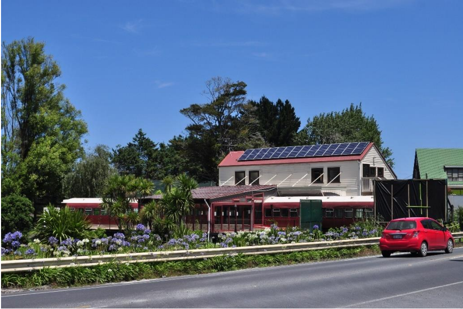
Figure 8-5: Railway carriages (017) next to SH16.
