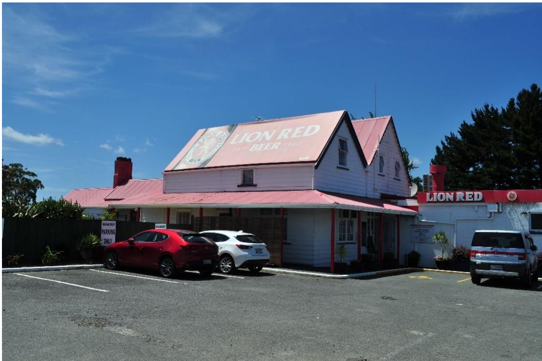
Figure 4-4: Main (pre-1900 core) buildings of the Huapai Tavern. Pre-1979 20 th century single-storey extensions to the right with 'Lion Red' sign (After Bader et al 2021)
