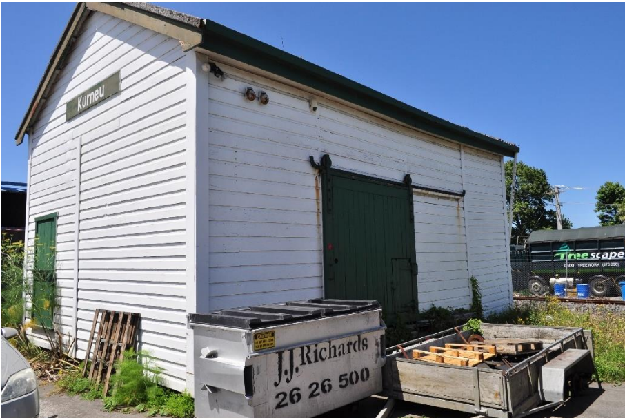
Figure 8-6: Railway shed (019) scheduled in the AUP;OP, next to the railway line.
