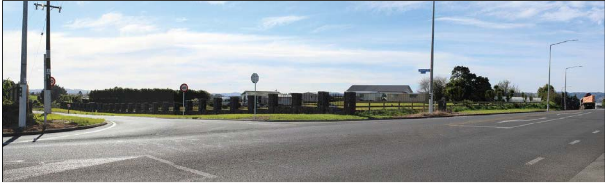
Figure 4: Corner of 8 Whangapouri Road at intersection. Source: Figure 7 of NoR: VP01 Before image, viewpoint from oncoming traffic opposite the site
