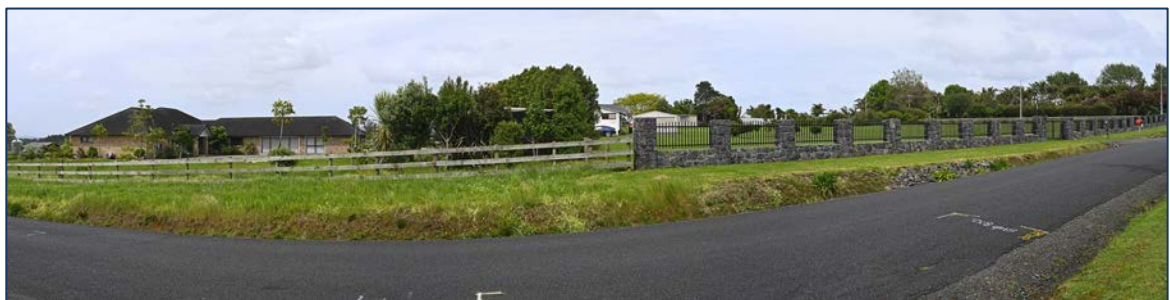
Looking towards the substation site from the previous driveway to 5 Whangapouri Road
