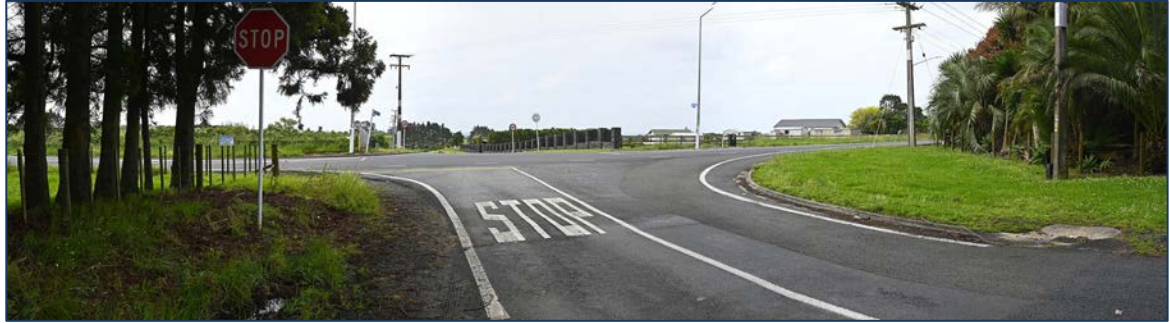
Looking towards the substation site from Bycroft Road across the intersection with Karaka Road
