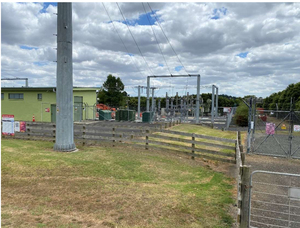
Figure 6: Existing substation at Whangarata Road, Tuakau.
