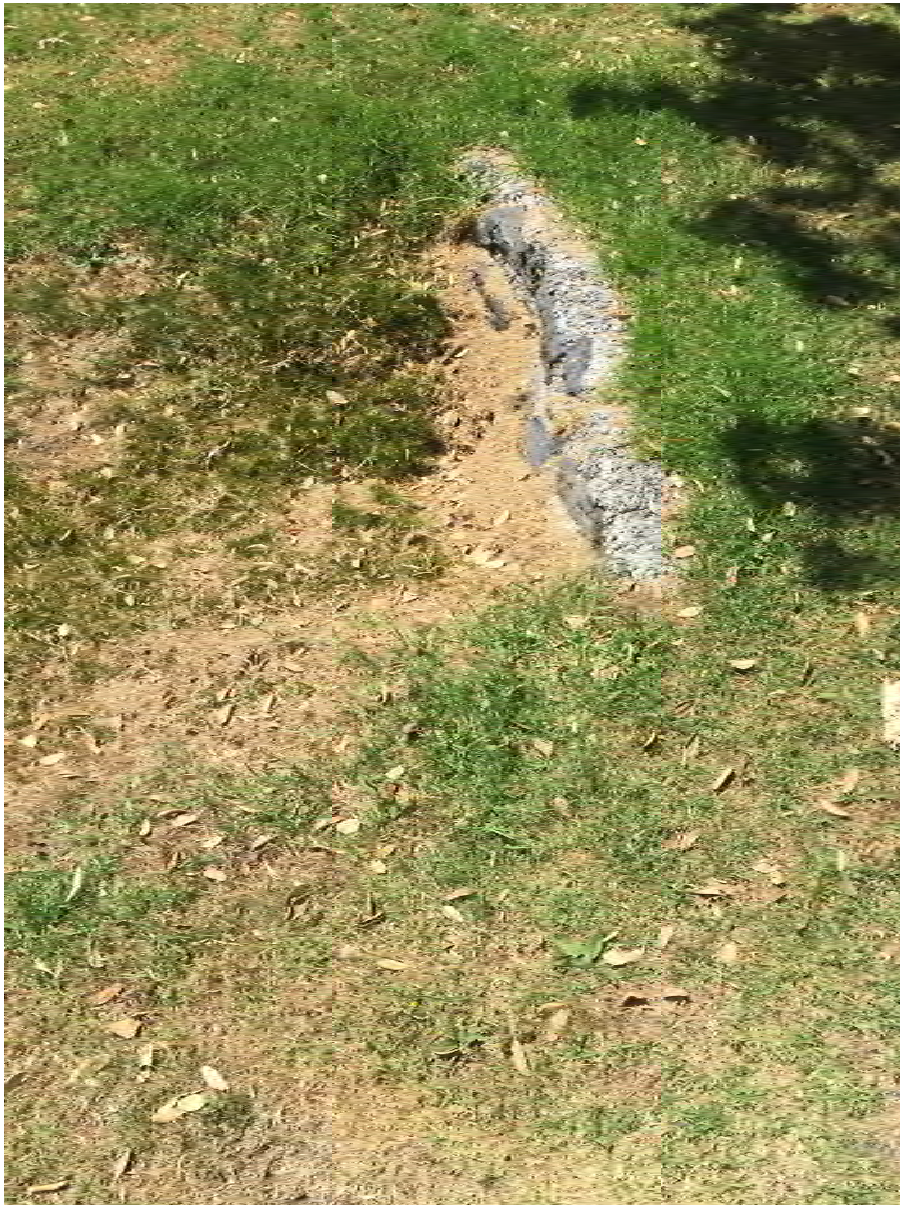
Open drain on North Eastern side of road.
