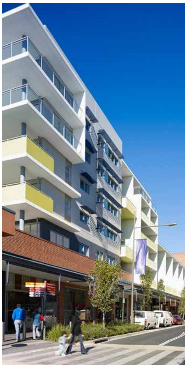
Rouse Hill Town Centre, Sydney - Example of high quality retail mainstreet with apartments above. (Photo supplied by Auckland Design Manual)
