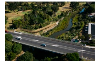
Cascades Road bridge showing the walkway connection down to the Cascades Walkway.
