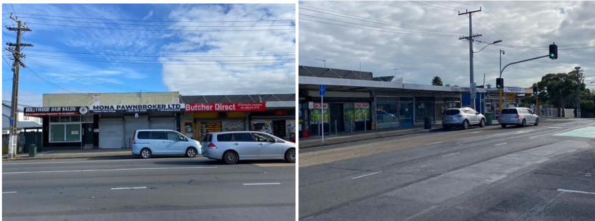
Figure 10: Puhinui Road business cluster (Puhinui Road opposite Ranfurly Avenue)
