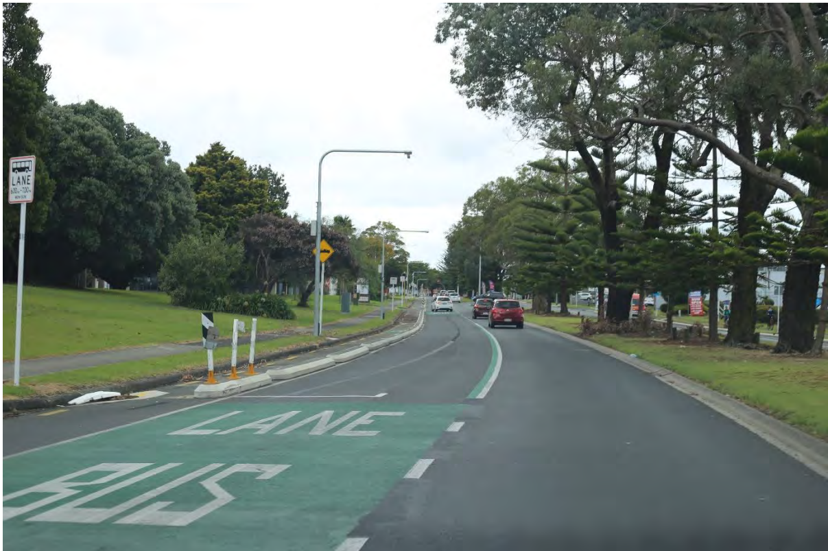
Figure 26: Lambie Drive north bound, north of Cavendish Drive
