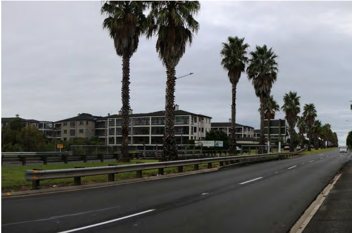
Figure 4: Metlifecare Dannemora, Retirement Village on the western side of Te Irirangi Drive
