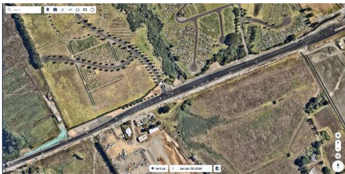
Figure 32. Large parts of the northern side of SH20B within NoR1a and NoR1b have been earth-worked and do not currently support indigenous vegetation or associated habitats.
