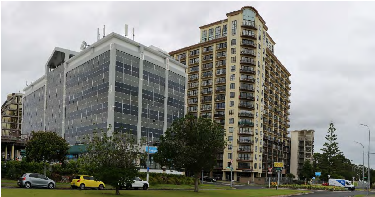
Figure 23: Western end of Ronwood Avenue with high rise apartments on the corner of Osterley Way and Hayman Park in the distance
