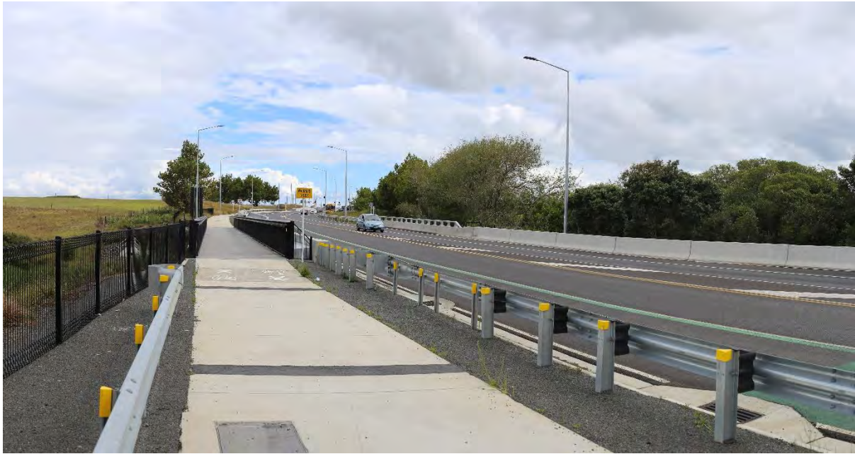
Figure 39: SH20B, bridge over Waokauri Creek, westerly view towards Auckland Airport
