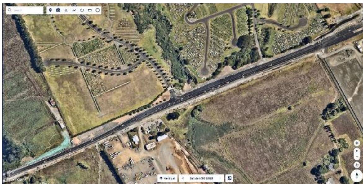
Figure 32. Large parts of the northern side of SH20B within NoR1a and NoR1b have been earth-worked and do not currently support indigenous vegetation or associated habitats.
