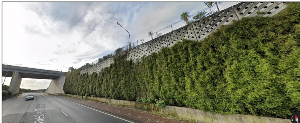
Figure 11 – Example of planted retaining wall on SH16 (Google streetview).
