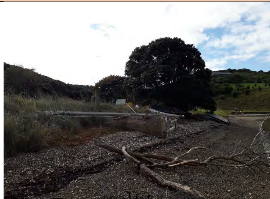
Looking east along northern portion of site
