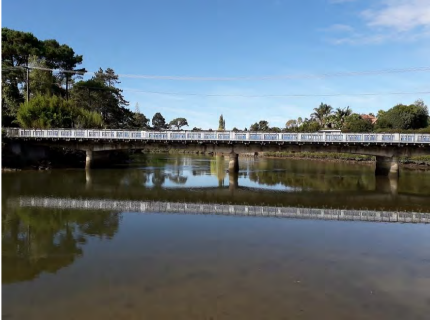
From within looking south towards Coatesville-Riverhead Highway Bridge
