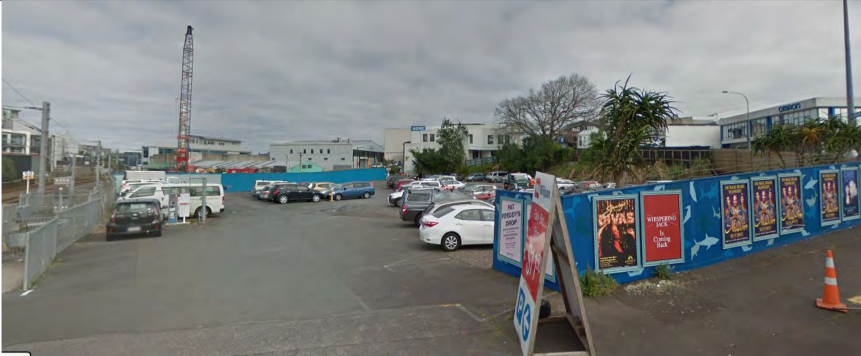
From Normanby Road Looking west across site
