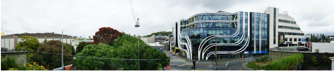
Mercury Energy Building – Submission #50 33 Broadway Trust (looking north)
