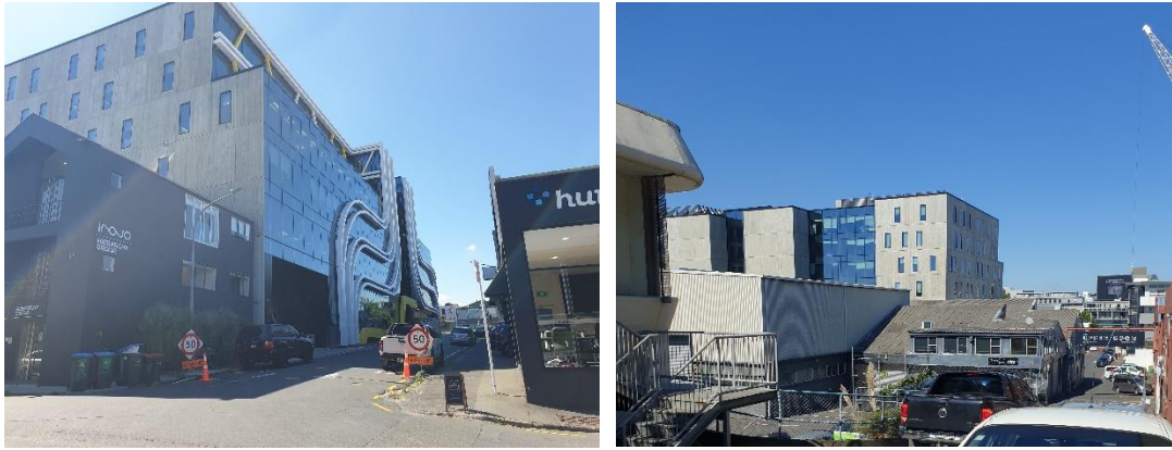
Photographs 26 & 27: View of Mercury Energy building at 4-10 Alma Street and 33 Broadway from Alma Street and north side of building behind plan change area and existing building at 13-15 Morgan Street. Source: Report Author
