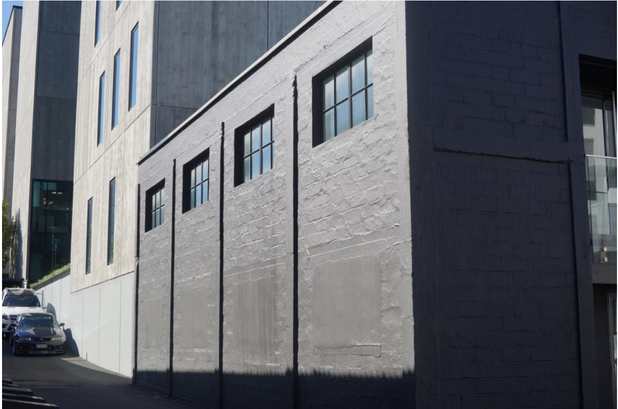
Figure 11: – Southern boundary of site - Service easement area off Clayton Street
