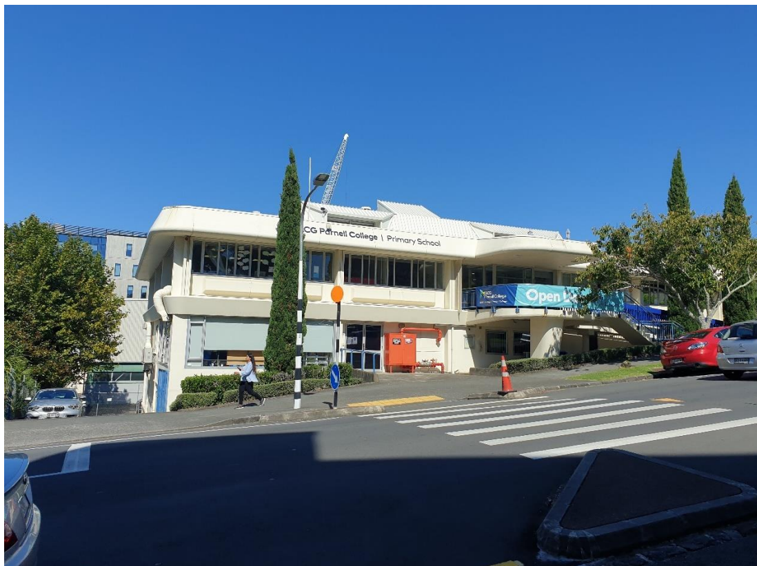
Photograph 9: View of building at 39 George Street (ACG Parnell College)
