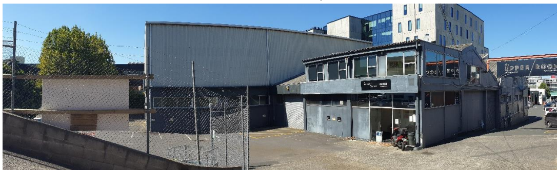
Photograph 3: View of existing buildings at 13-15 Morgan Street (to rear of 39 George Street) Source: Report Author
