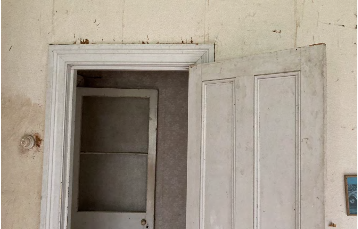
Figure 2. Original four-panel villa door and architraves. Beyond is the hall door minus original glazing and all but one glazing bar.
