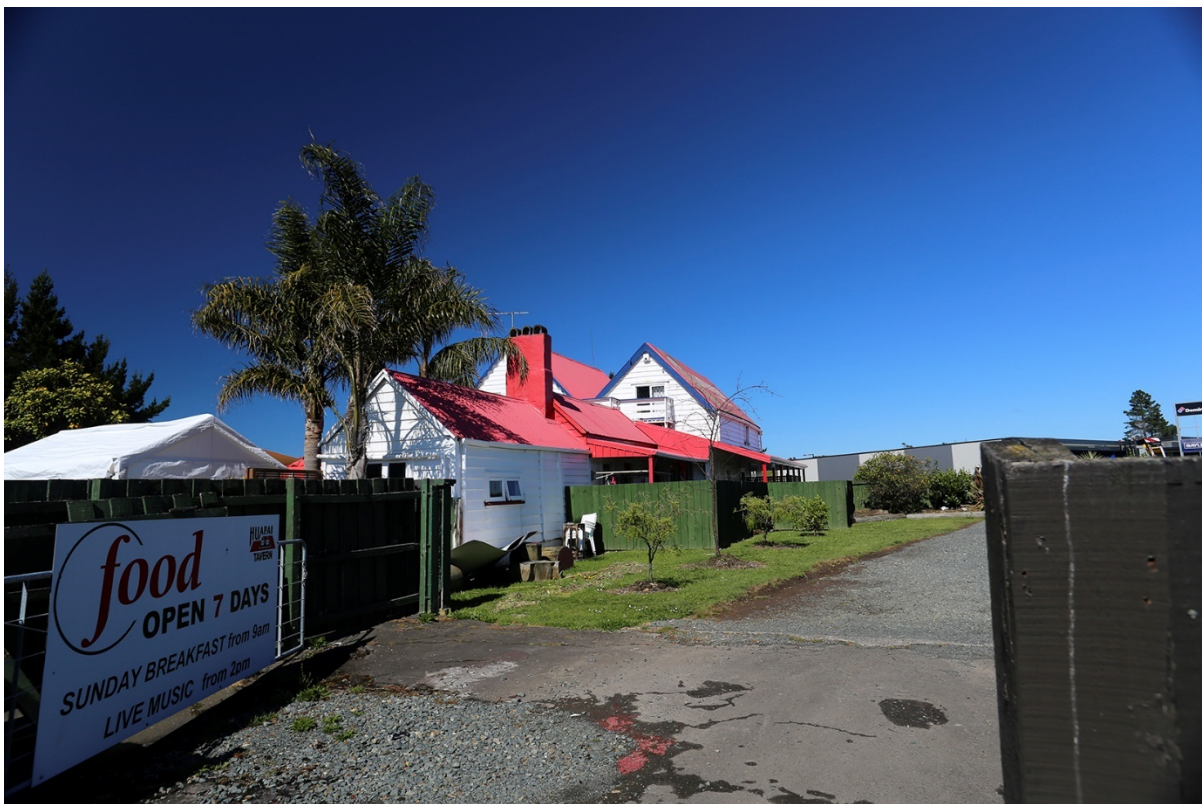
Figure 20: Huapai Tavern east elevation showing single surviving chimney (centre). Photo: Rachel Ford (31/10/20108)
