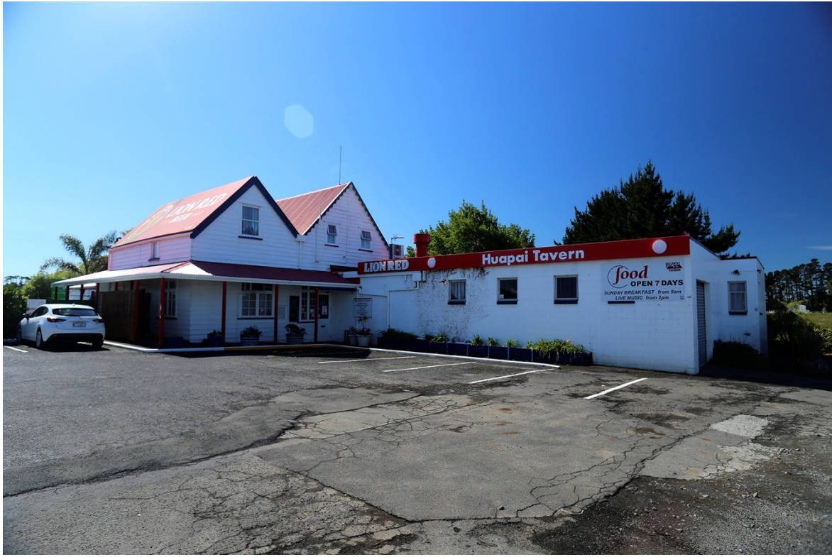
Figure 19: Huapai Tavern north and west elevation with 1970s addition to the right. Photo: Rachel Ford (31/10/2018)
