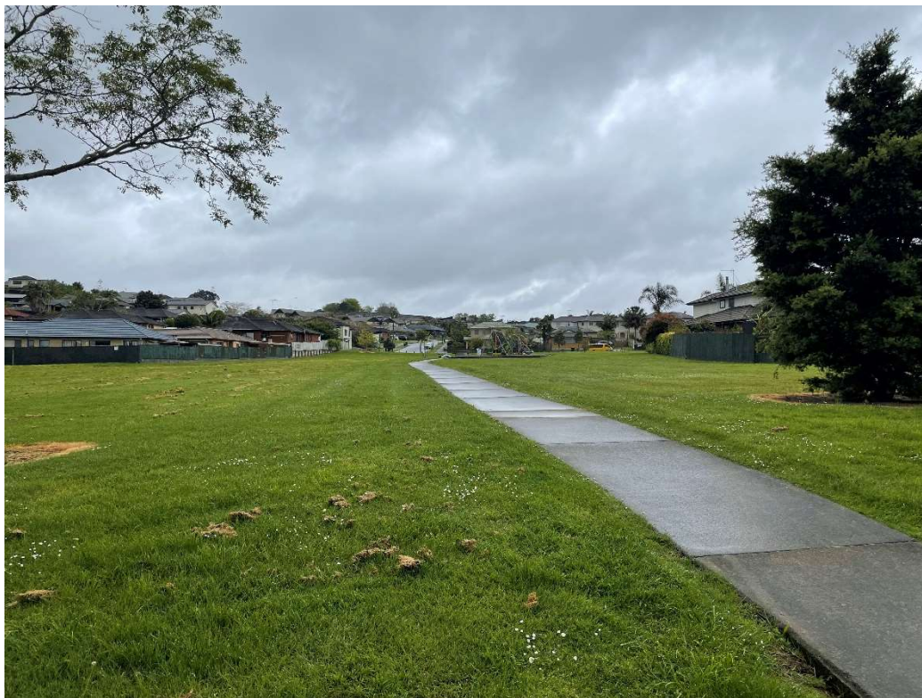
Figure 37 - Existing Path within Alfriston Park, as viewed from Alfriston Road, looking north. Source: Site Visit Photo
