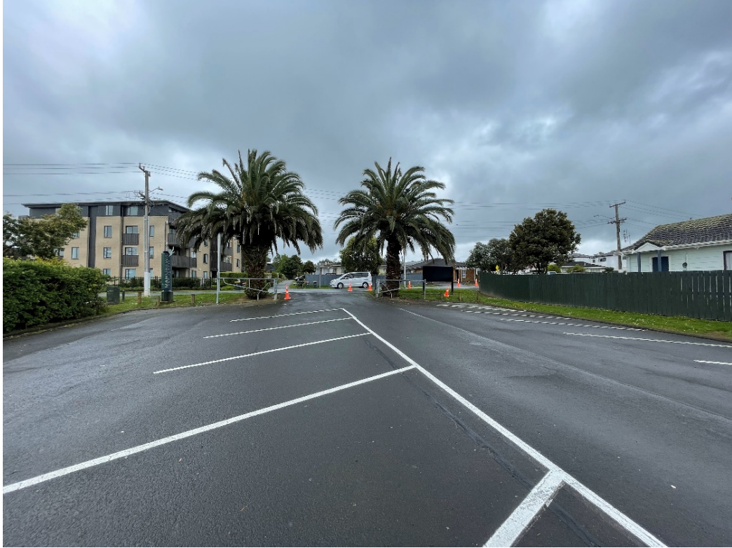
Figure 28 - Gallaher Park car parking area looking north toward Alfriston Road. Source: Site Visit Photo
