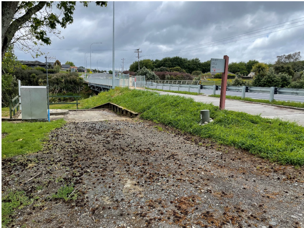
Figure 19 – Image showing area of proposed bridge retaining support on the western side of Slippery Creek Reserve adjacent to Great South Road. The utility cabinet on the right of the image may need to be relocated. Source: Site Visit Photo
