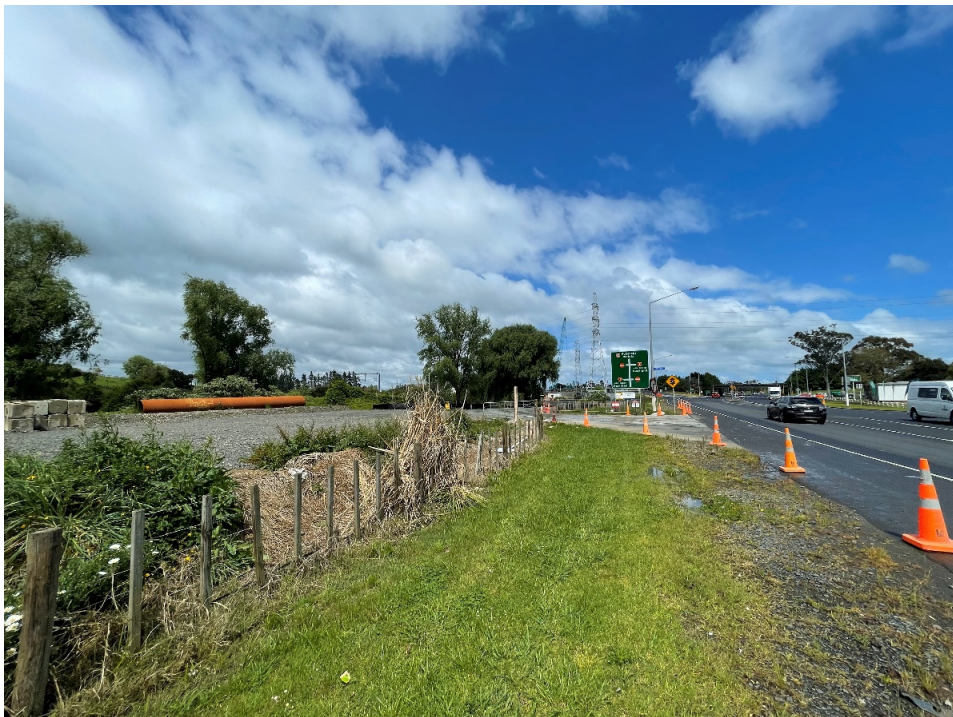
Figure 21 - Karaka Reserve, looking south-west from Great South Road, showing metalled laydown area on site, construction material, and lack of any obvious open space character or utilisation. Source: Site Visit Photo
