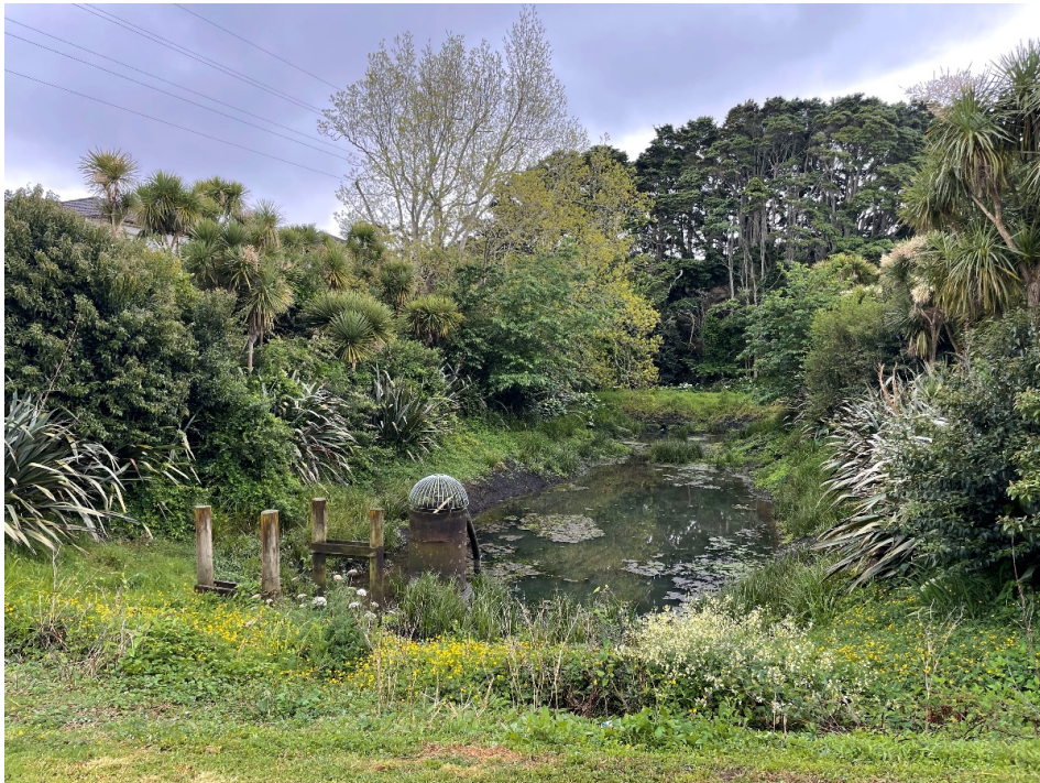
Figure 32 - Stormwater detention pond within Index Place Reserve. Source: Site Visit Photo
