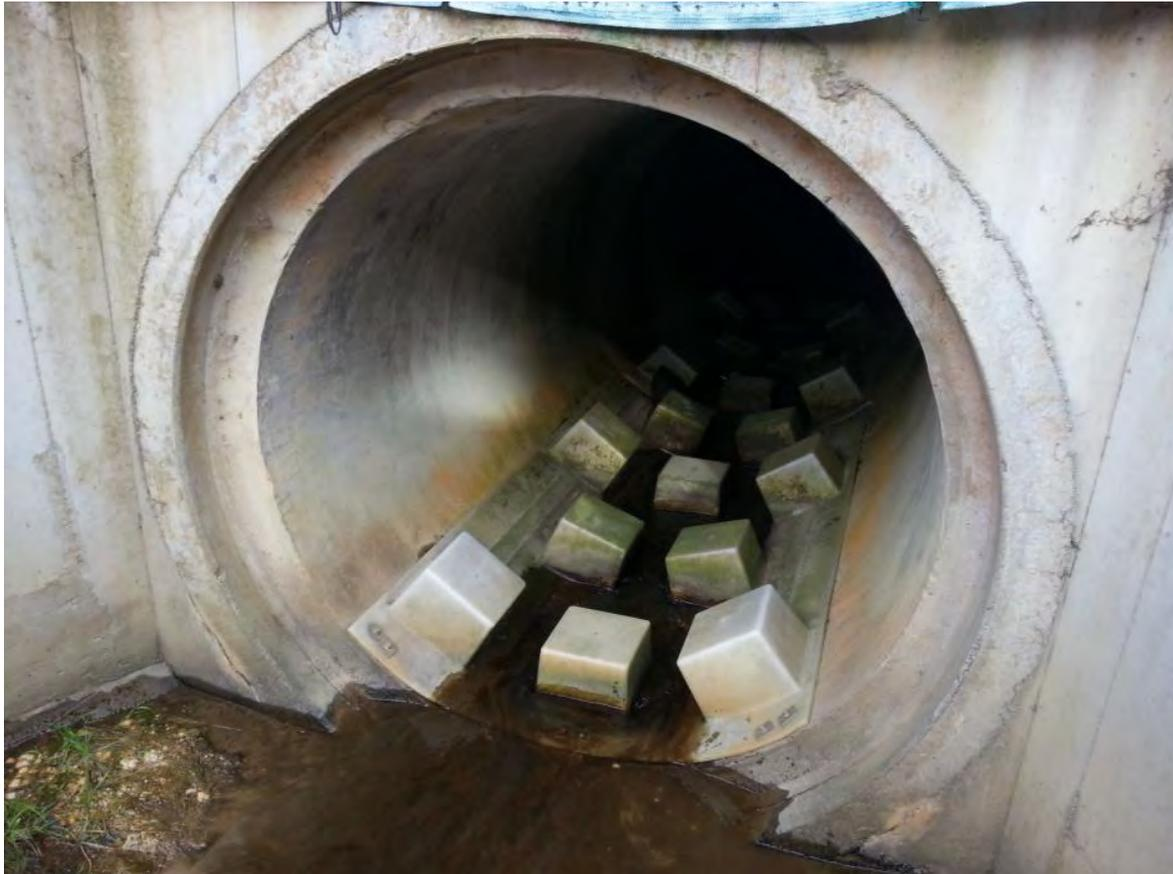
Figure 4–8: Baffle type fish passage installed at Waiwera
