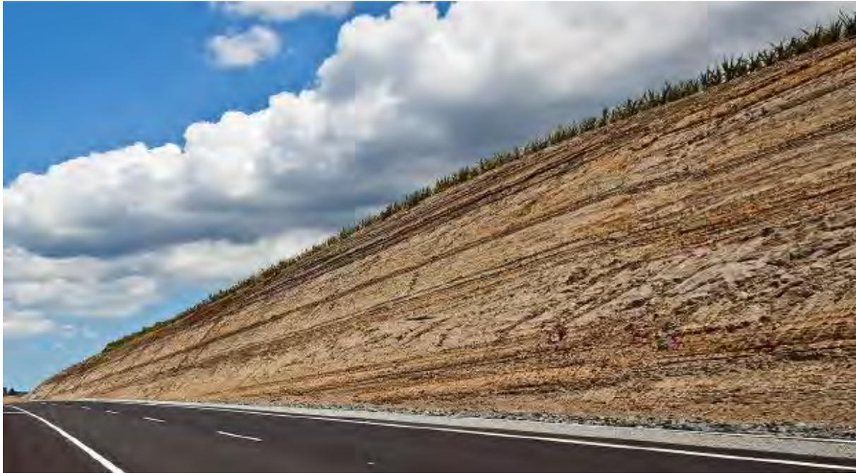
Figure 4-7: Indicative cut face batter (possible for cuts within the plantation forestry area)
