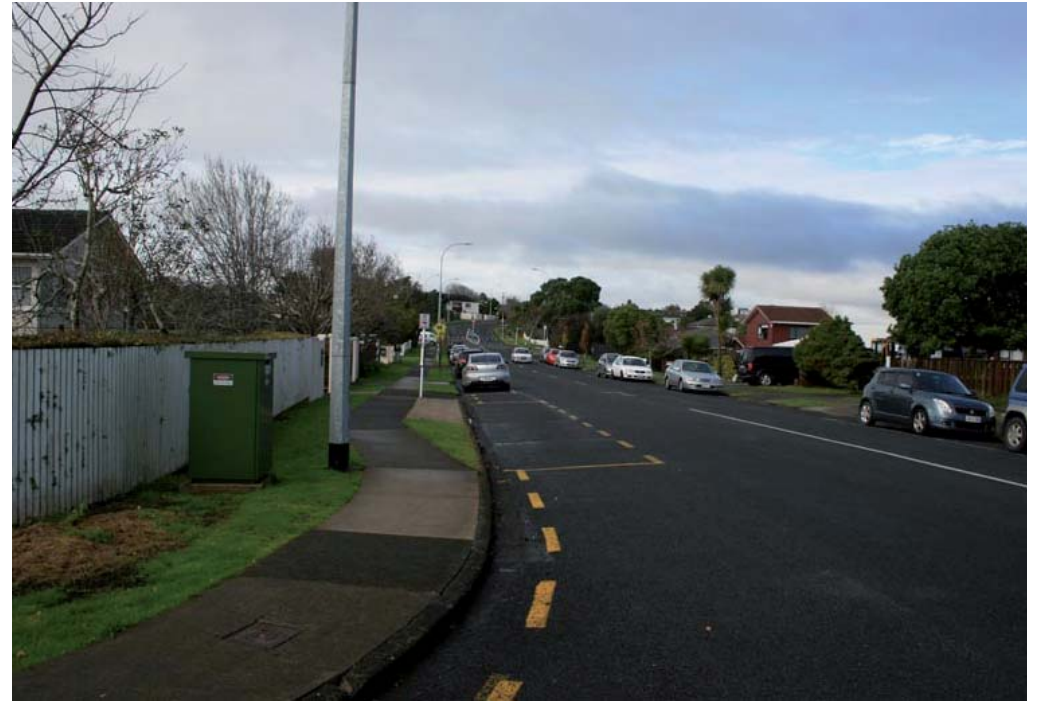
Image 17: Sandspit Road from Reydon Place looking south
