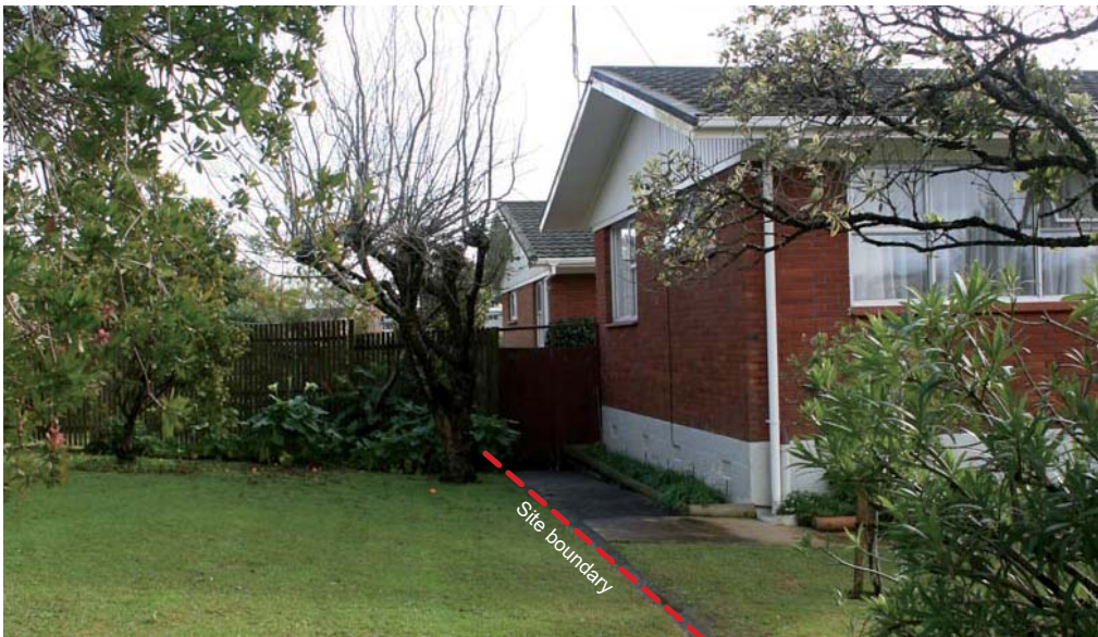
Image 29: Western facades of dwellings at 6 and 6a Reydon Place very close to the boundary
