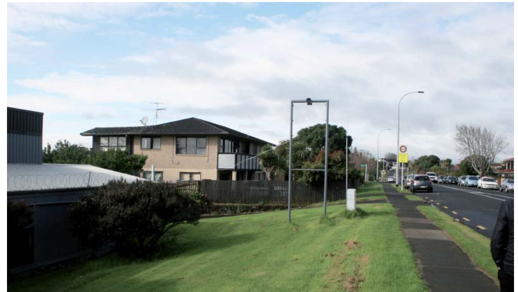
Image 25: View along the front boundary with workshop to left and main dwelling at 40 Sandspit Road
