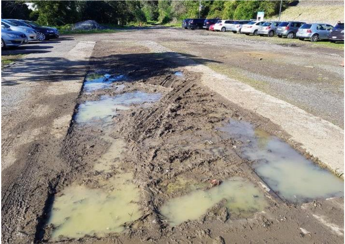
Figure 17. Probably the infilled remains of an inspection pit within the former workshop
