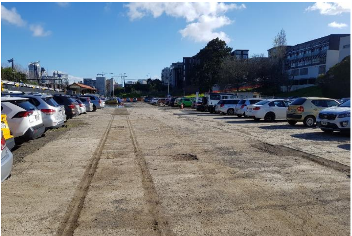
Figure 16. Looking north showing remnant rail tracks formerly in the workshops
