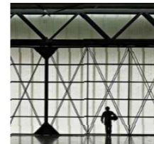
St.01 - Structure Exposed steel columns, trusses and bracing.
