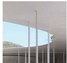
St.01 - Steel Columns and canopies.
