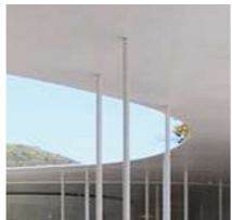
St.01- Steel Columns and canopies.
