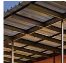
St.01 - Structure Exposed steel columns and roof framing.
