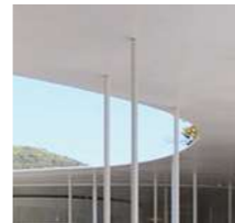
St.01 - Steel Columns and canopies.
