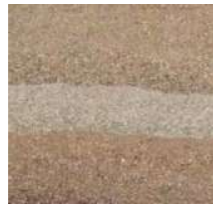
W.01 - Rammed Earth Rammed earth with local sandstone.
