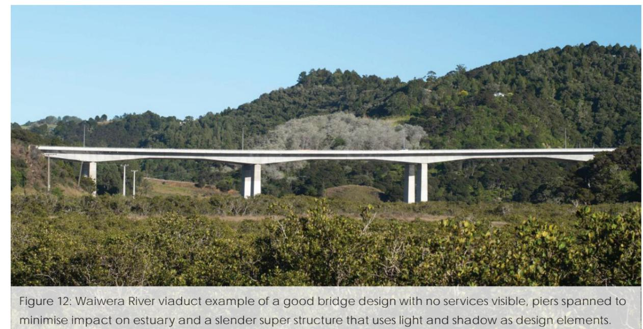
Figure 12: Waiwera River viaduct example of a good bridge design with no services visible, piers spanned to minimise impact on estuary and a slender super structure that uses light and shadow as design elements.
