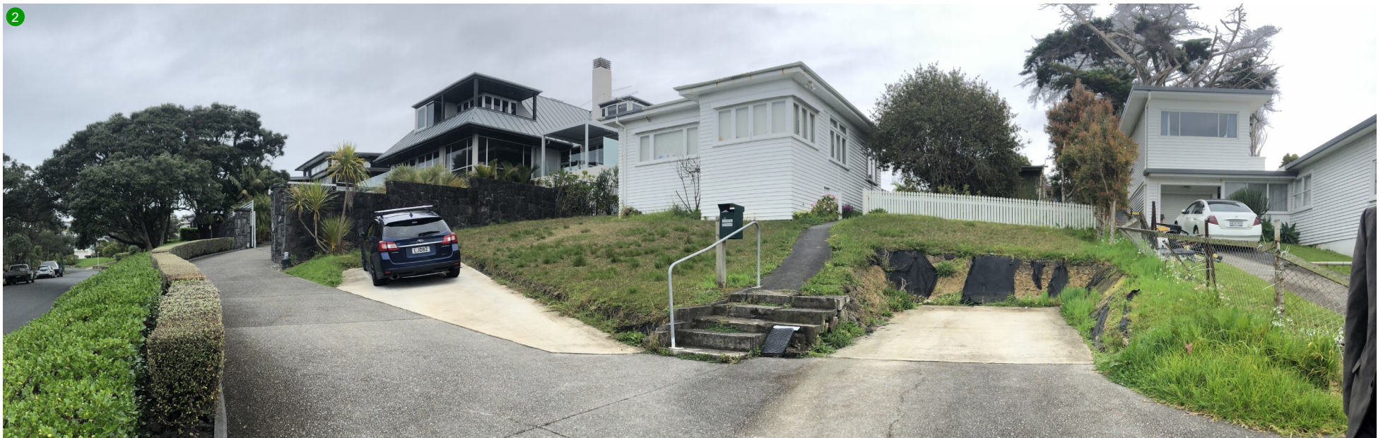
ABOVE FIG. 2-5: The Site viewed from Whitby Crescent, with the slip road providing access to adjacent 21 Whitby Crescent in the foreground.
