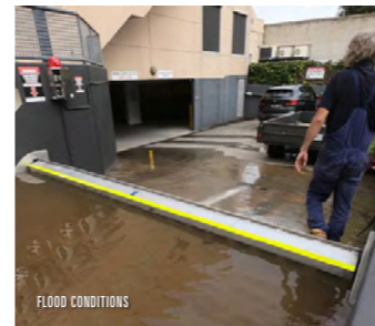
^ Pictured above is the Floodfree Passive Tilting Flood Barrier which self-deploys as water levels rise.
