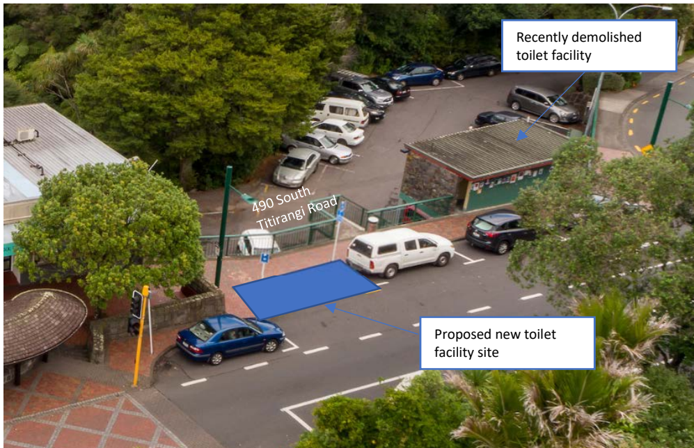
Figure 1: Historic drone image showing location of the proposed new toilet facility site (Option B) and the recently demolished toilet facility outside 490 South Titirangi Road
