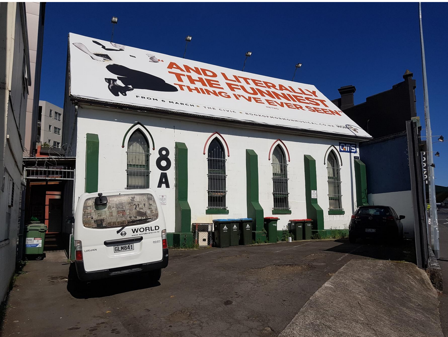
Figure 8 Photograph of roadside (western) wall of building Historic Site
