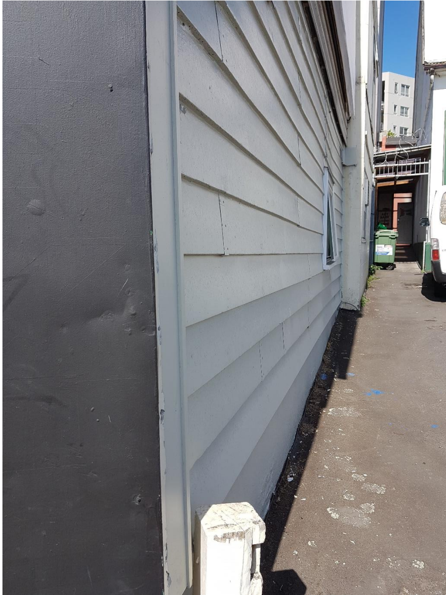
Figure 4 Photograph along southern boundary wall of Subject Site
