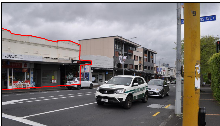
Character supporting building (outlined in red) immediately south of the subject site. Source: DPA Architects, 2019
