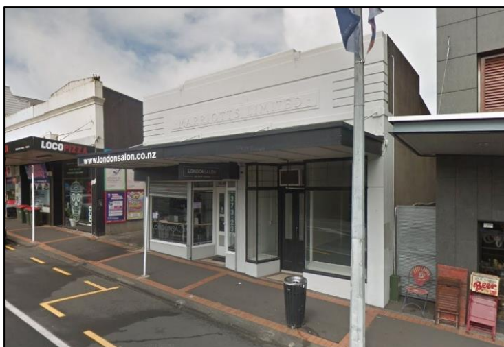
Building composition with parapet wall and glazed shop frontage promoting street activation. Source: Google maps
