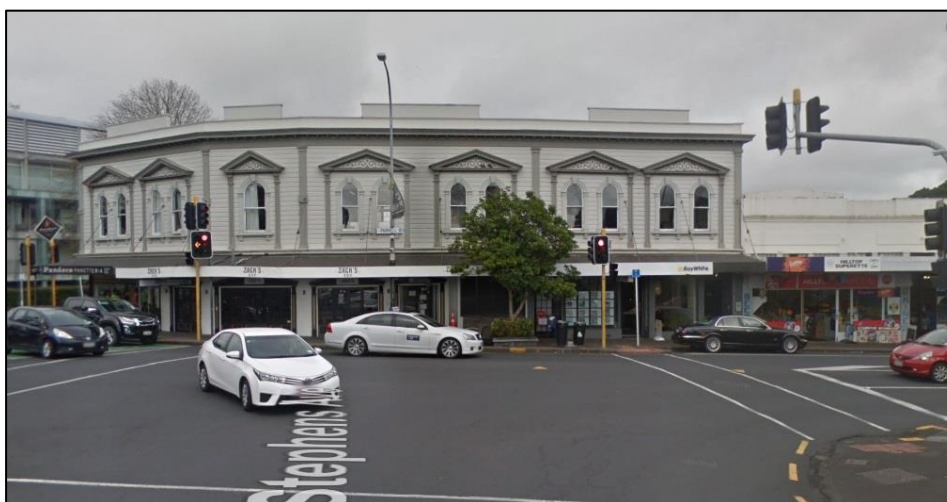
Timber Italianate building on the southern-most corner of the special character area known as the Kemp department store. Source: Google maps, street view.
