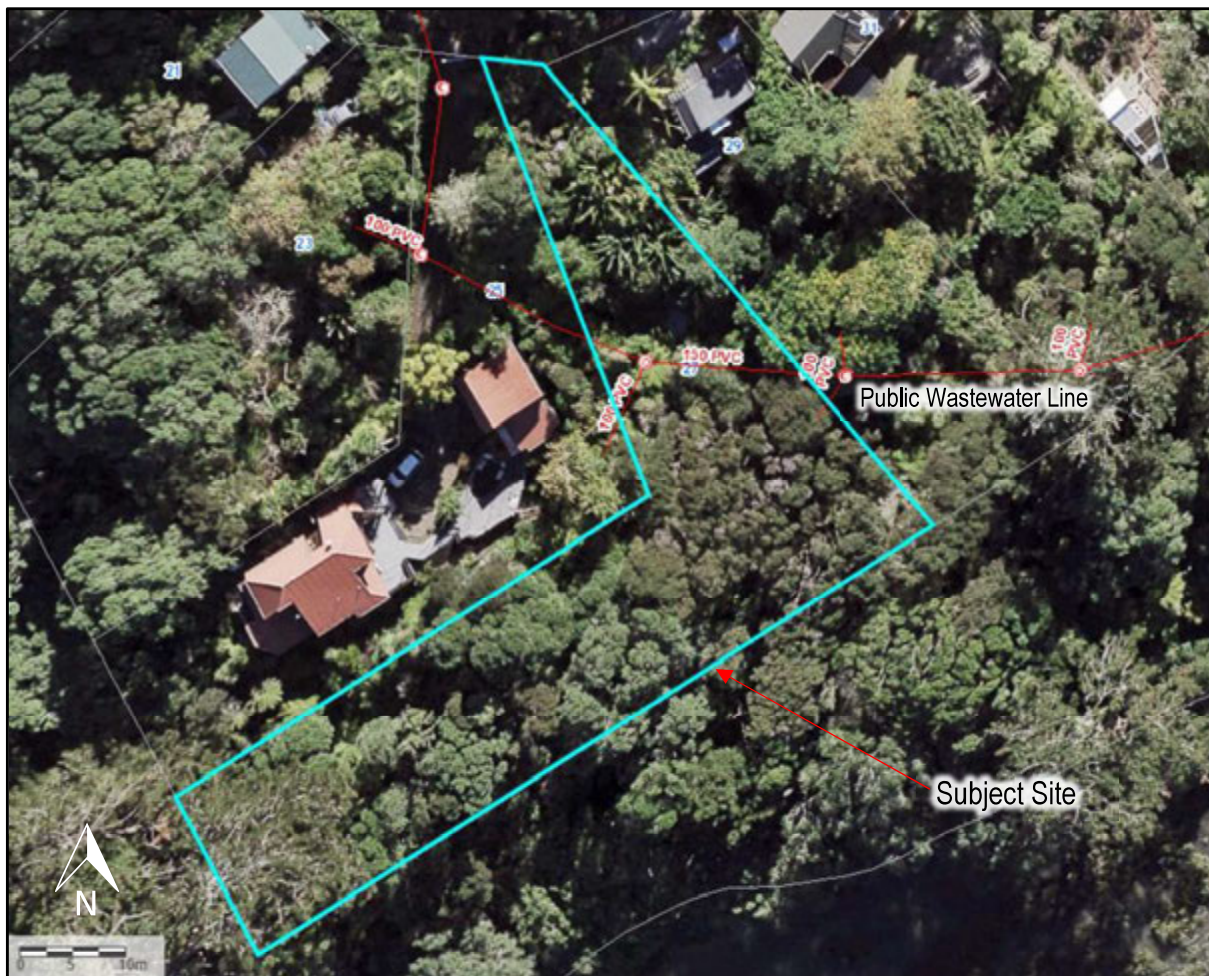
Figure 1: Aerial Photo (Auckland Council GeoMaps)
