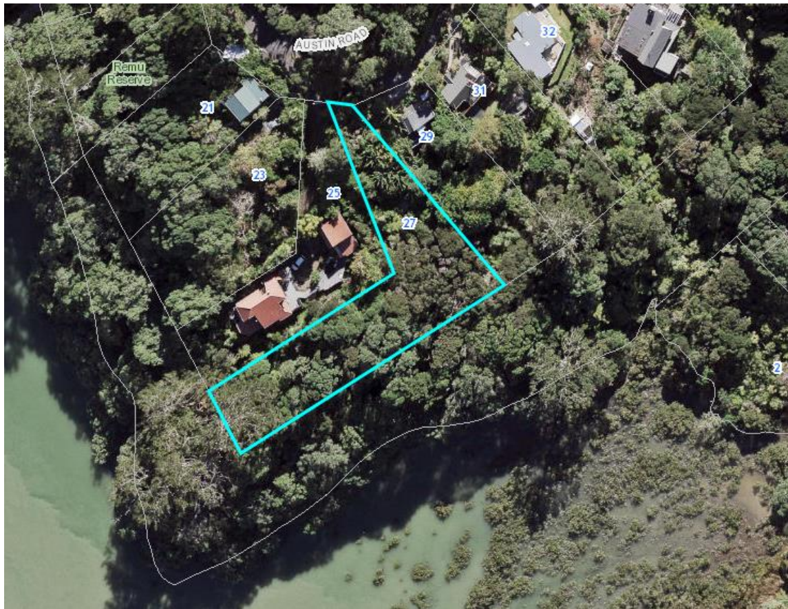
Figure 1: Aerial photo of subject site, 27 Austin Road, Greenhithe.
