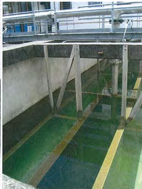
Working gravity sand filter at the Huia Plant
