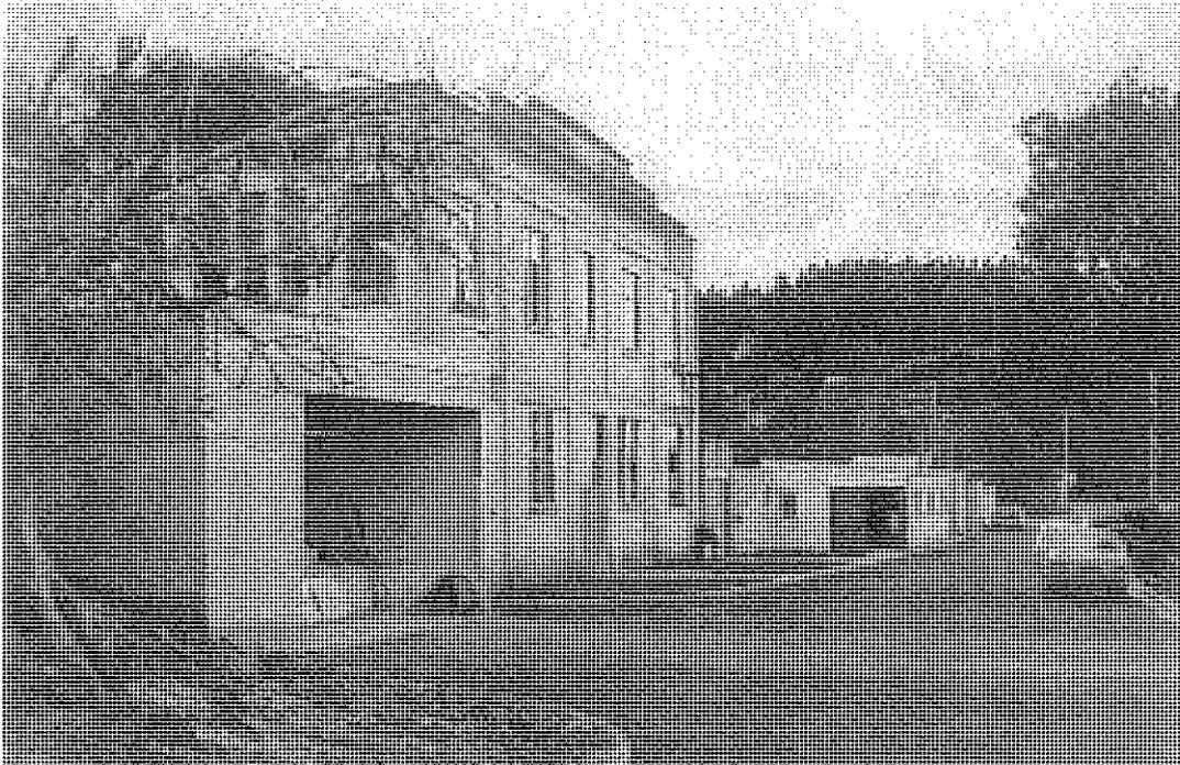
Nihotupu Water Filter, operational in 1970s with hand pressure tanks and stone bedded, prior to construction of west addition and reservoir. Photo: Watercare archives
