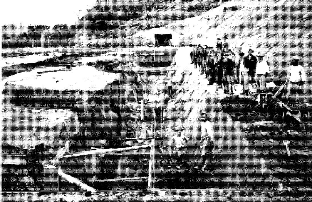
View of Nihotupu Water Filtration Chambers under construction, showing along side placement of bedlogs.
