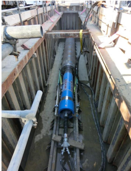
Figure 25. Photograph of indicative pipe hammering set up (Source: Brian Perry Civil)
