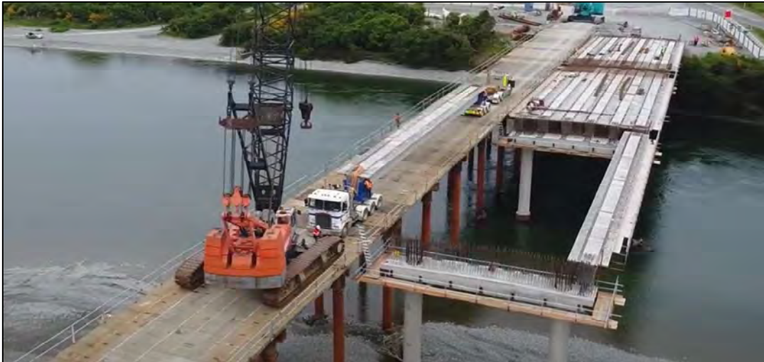
Figure 4-20 An Example of Typical Temporary Staging within the CMA
