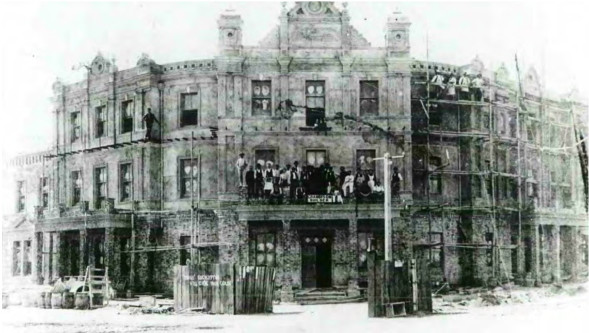
The Esplanade building under construction (~1902) 25
