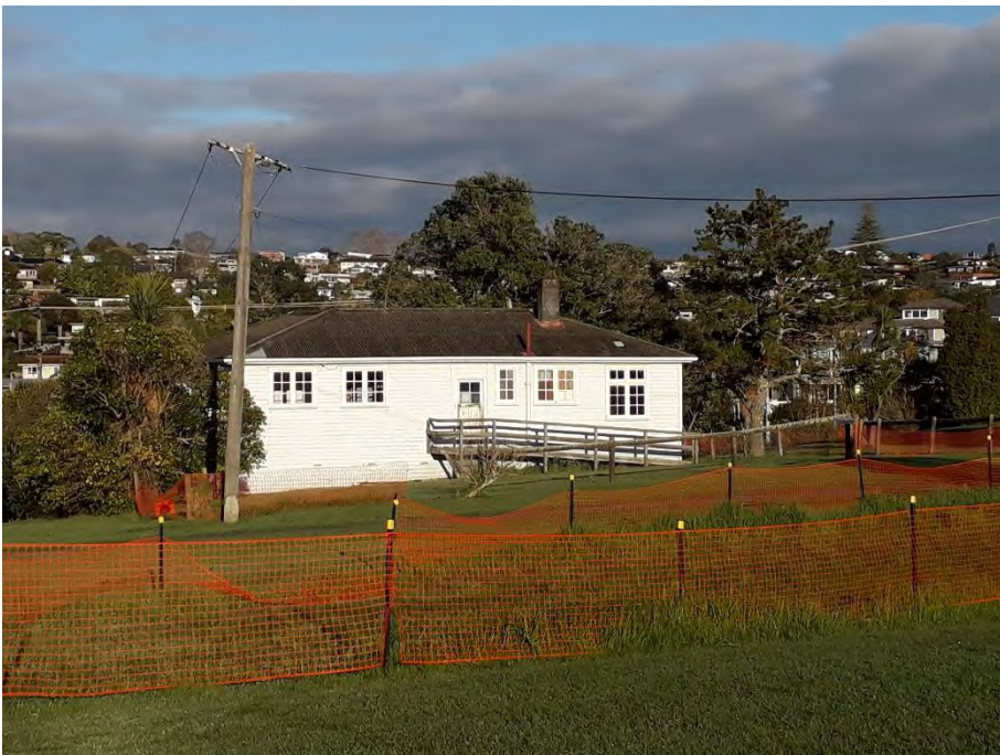
Former barracks/recreation building.
