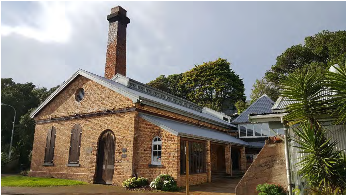
Figure 1: Pumphouse (Auckland Council; 8 July 2020)
