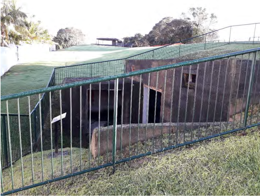
Former engine room
