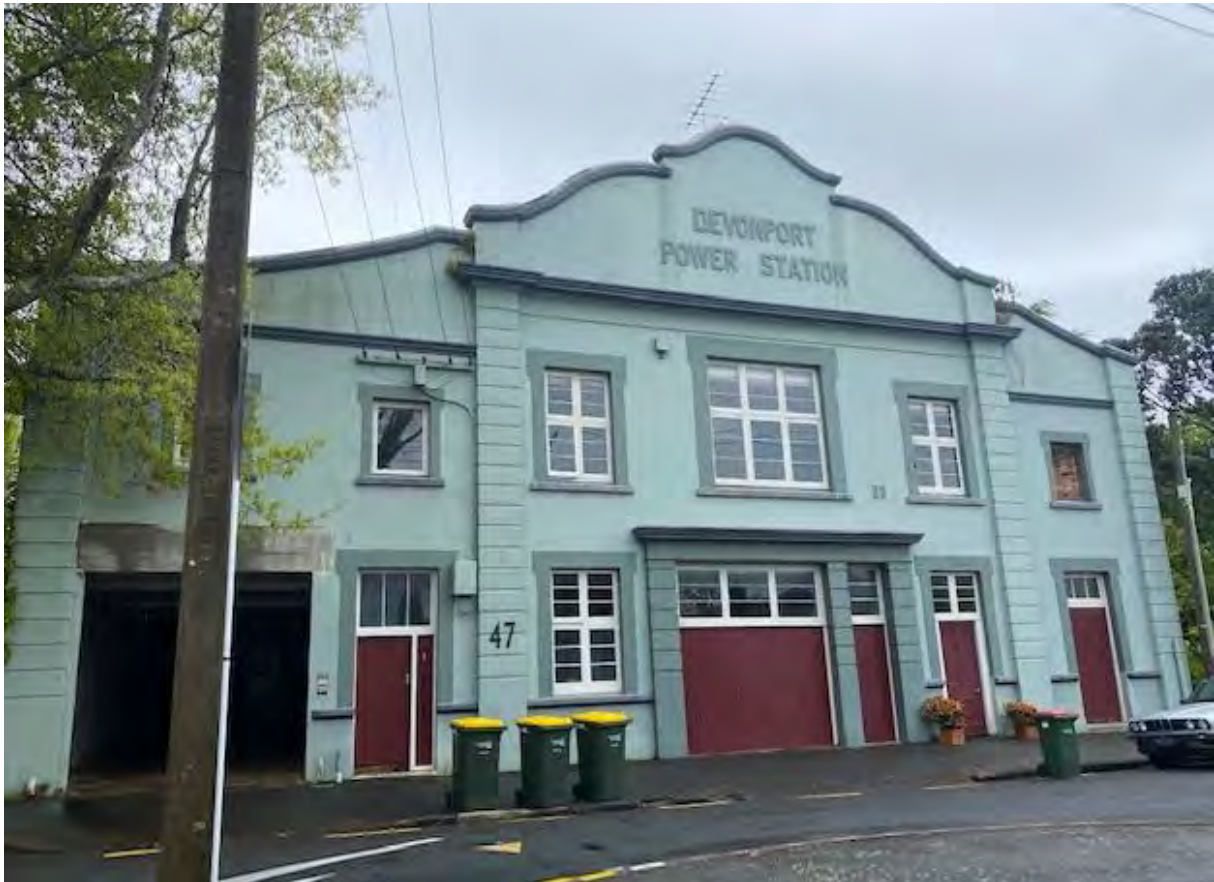
Figure 1: Devonport Power Station (former). Auckland Council, October 2020
