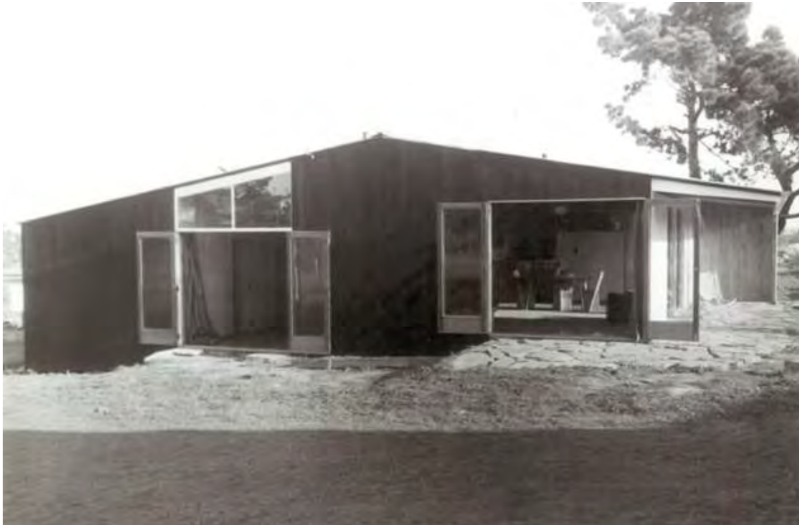
Figure 1: First House during its construction. 1
