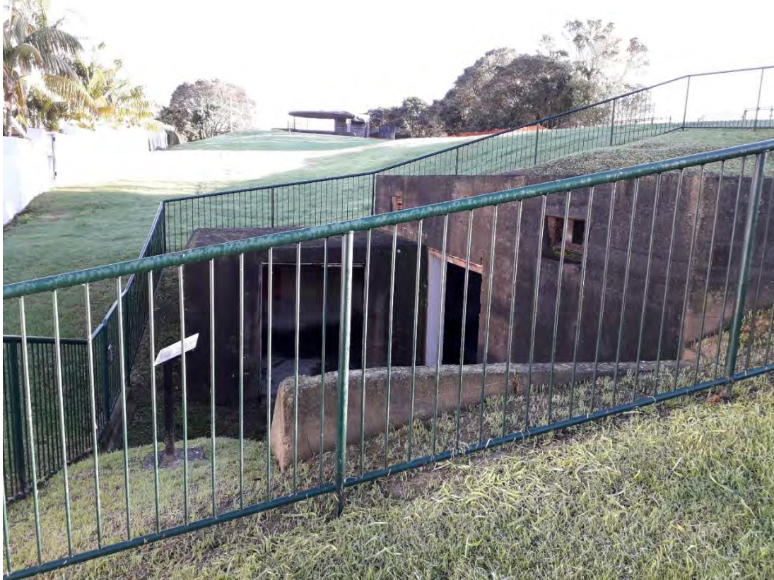
Figure 1: Castor Bay Battery complex engine room (David Bade, Auckland Council, 21 July 2020).
