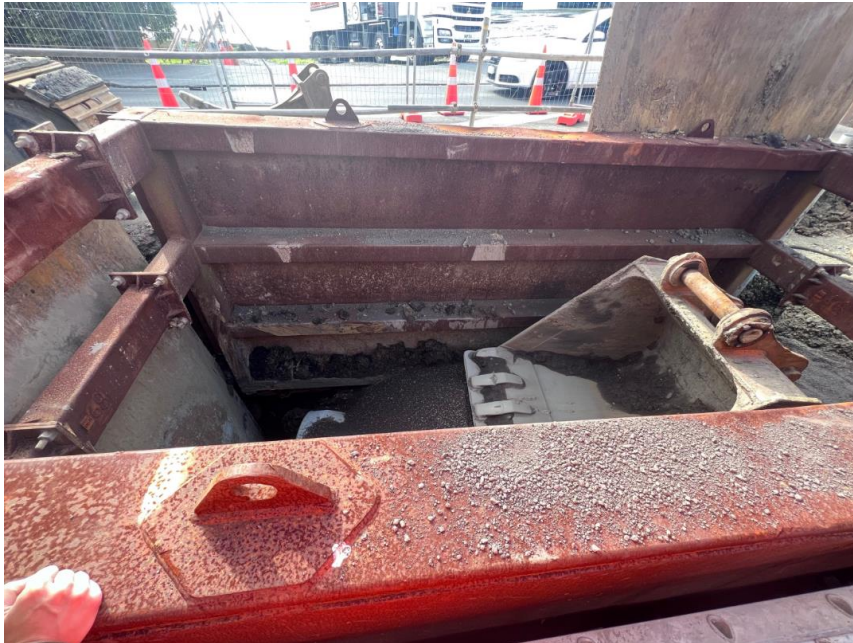
Figure 24. Example of open trenching using trench shields (Photograph: Tingran Duan, 2 September 2022)
