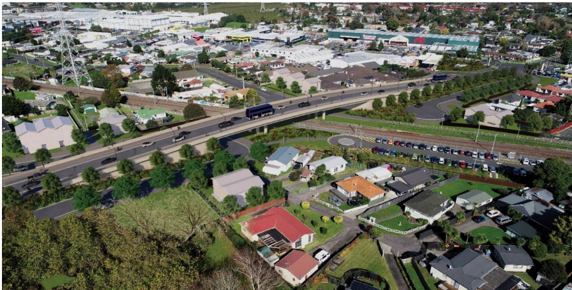
TAKA STREET GRADE SEPARATION AERIAL VIEW LOOKING SOUTH - JUNE 2023
