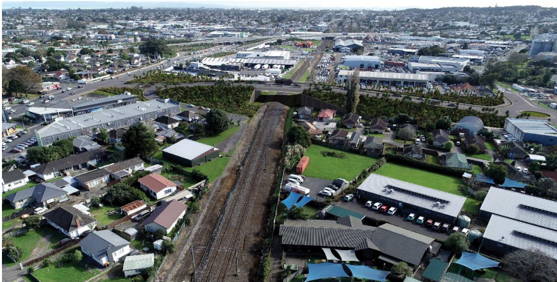
MANUIA ROAD GRADE SEPARATION AERIAL VIEW LOOKING NORTH WEST (WITH LOW PLANTING)
