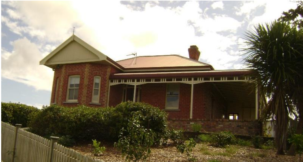
Figure 12: 19 Longbush Road – view of western elevation (photo by Jean Keay, 27 July 2020).
