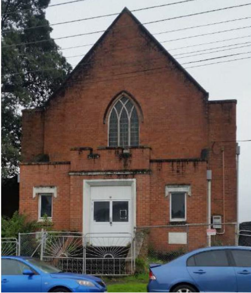
Figure 3: The former St Andrews Sunday school hall from an image taken in 2016 by Lilli Knight (Conservation Plan, Burgess, Treep & Knight).
