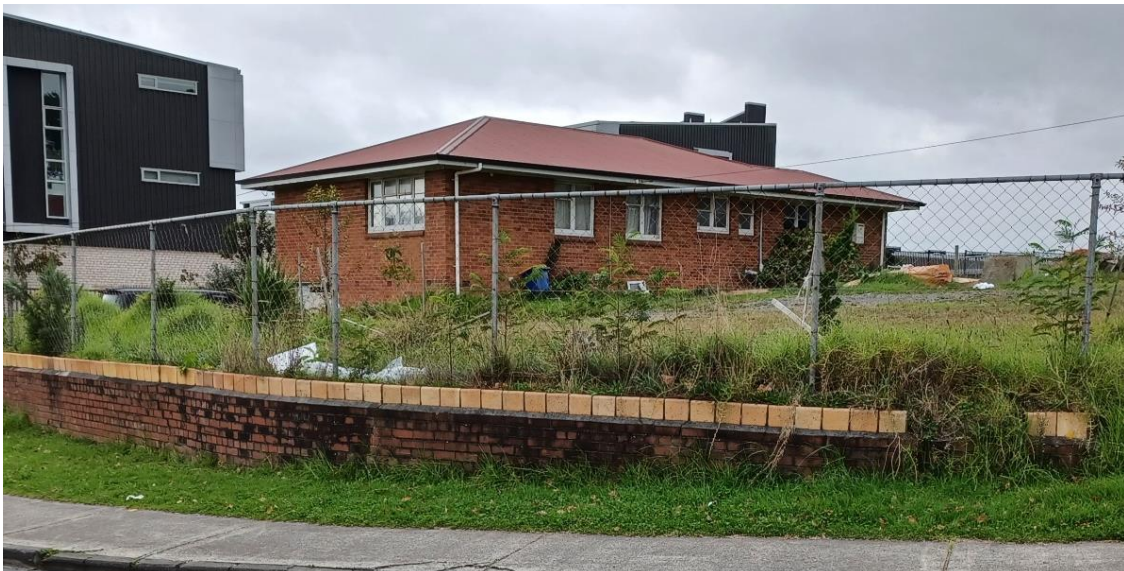
Figure 4: The former manse (Auckland Council, May 2022).
