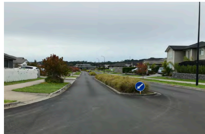
Central swales in Riverhead Point Drive
