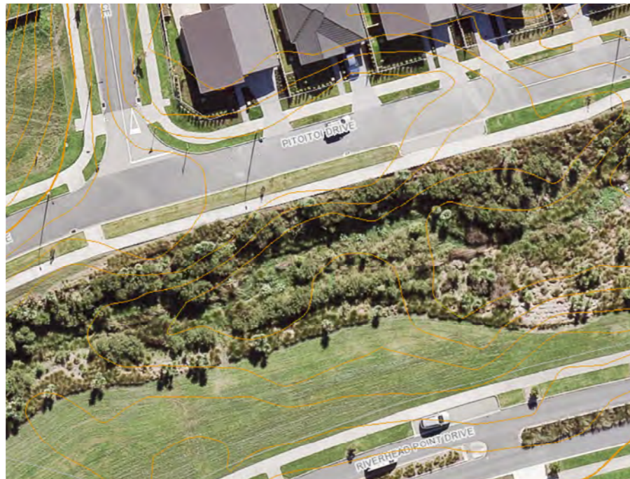
drainage corridor/swale along Riverhead Point Drive
