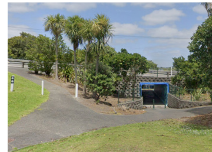
SH1 underpass off Kelgray Place through to Rodney College
