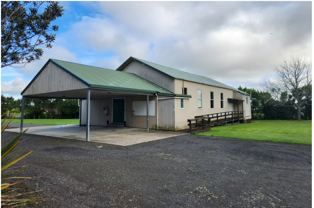
Figure 5-13 View northwest of Ramarama Hall
