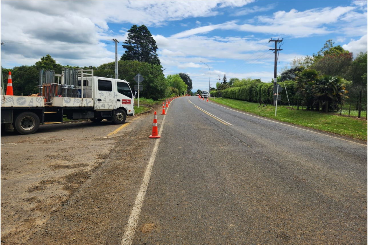
Figure 5-19 View west along Great South Road near St Stephen's School entrance.
