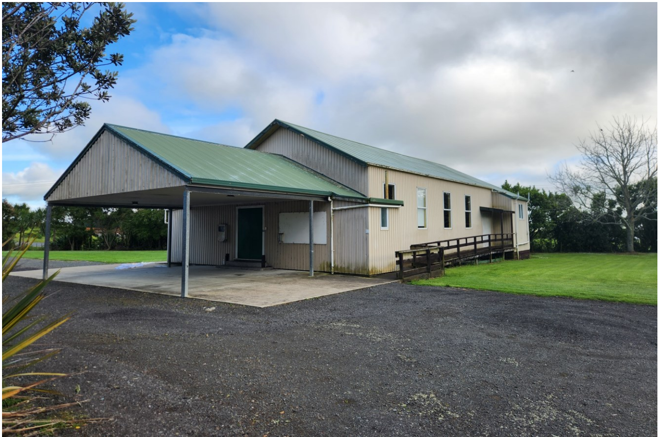
Figure 5-13 View northwest of Ramarama Hall
