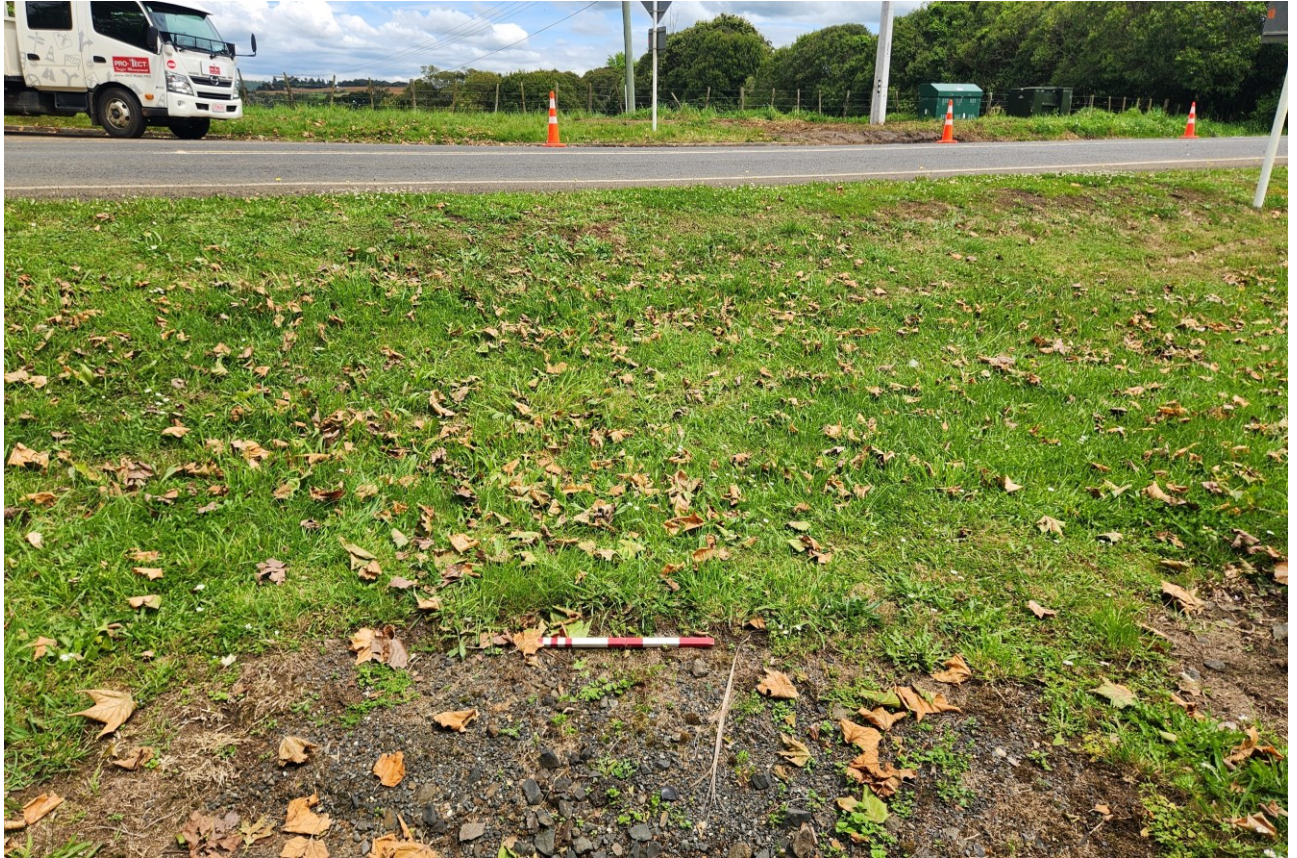
Figure 5-18 View south across Great South Road from drain to the unmodified portion of the creek. This is the suspected route of the culvert. Photo scale = 0.5 m.
