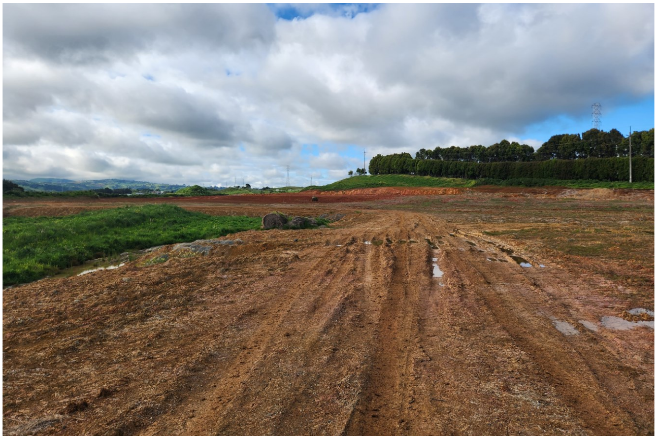
Figure 5-21 View south of Property 2 showing area recently cut with motor scraper.
