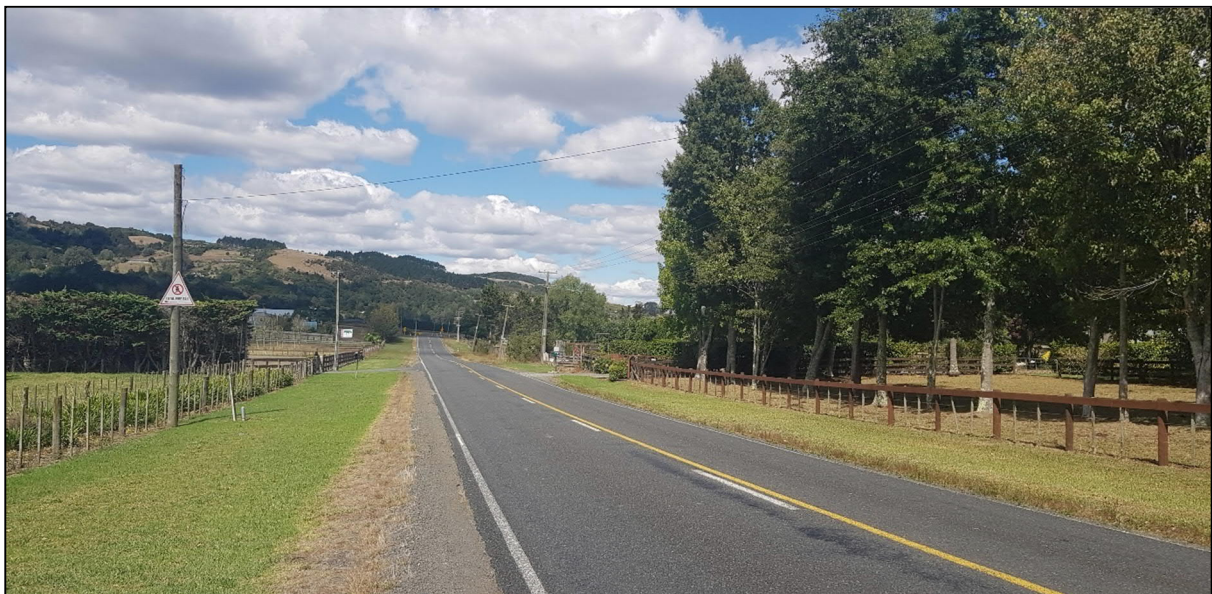
Figure 8-2. Waihoehoe Road, facing east.
