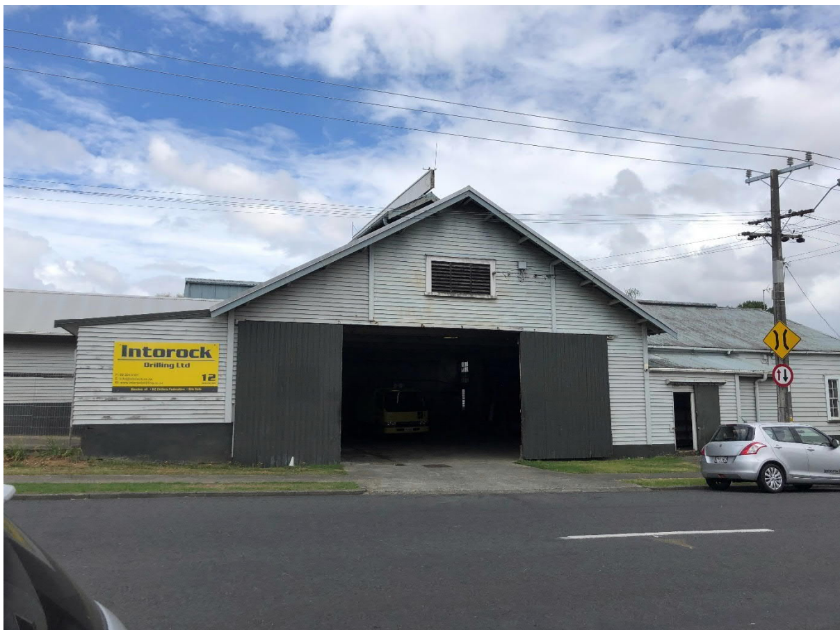
Figure 7-21. The Former Drury Creamery and Casein factory
