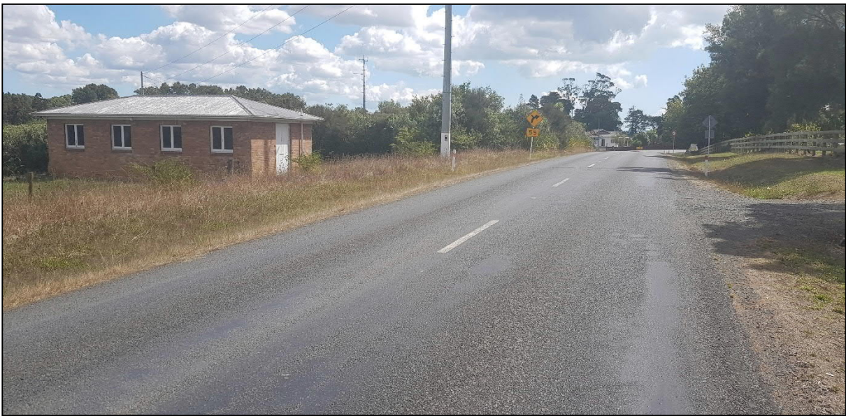
Figure 9-3. The 1940s Utility building, facing west.
