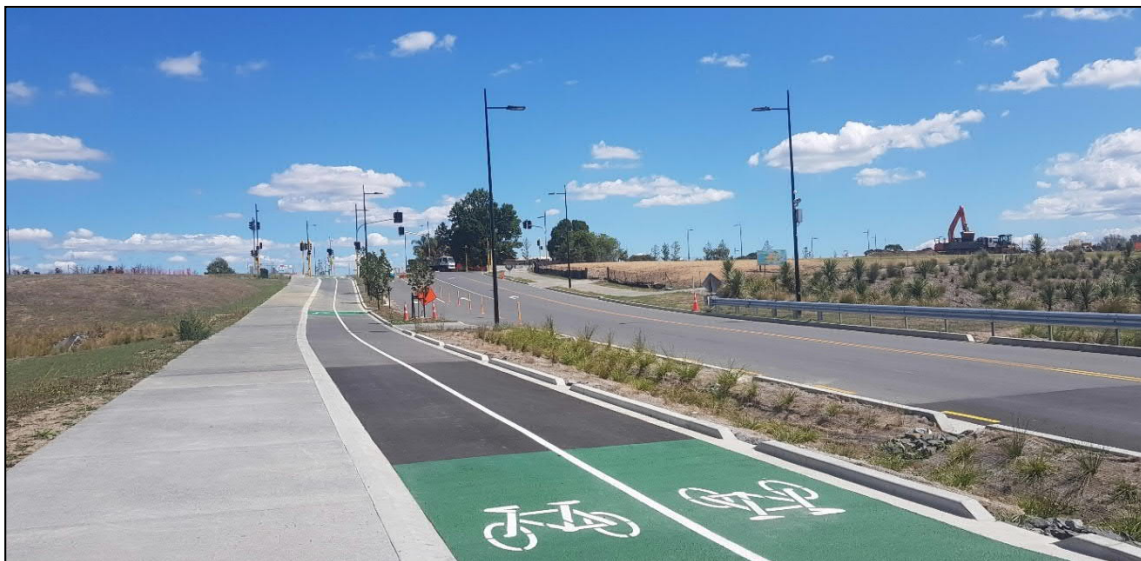
Figure 7-7. Bremner Road upgrade, facing west.
