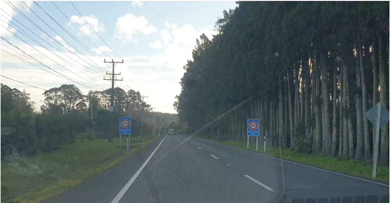
Figure 6: Typical layout of Riverhead Road (shown west of Coatesville-Riverhead Highway, looking west)
