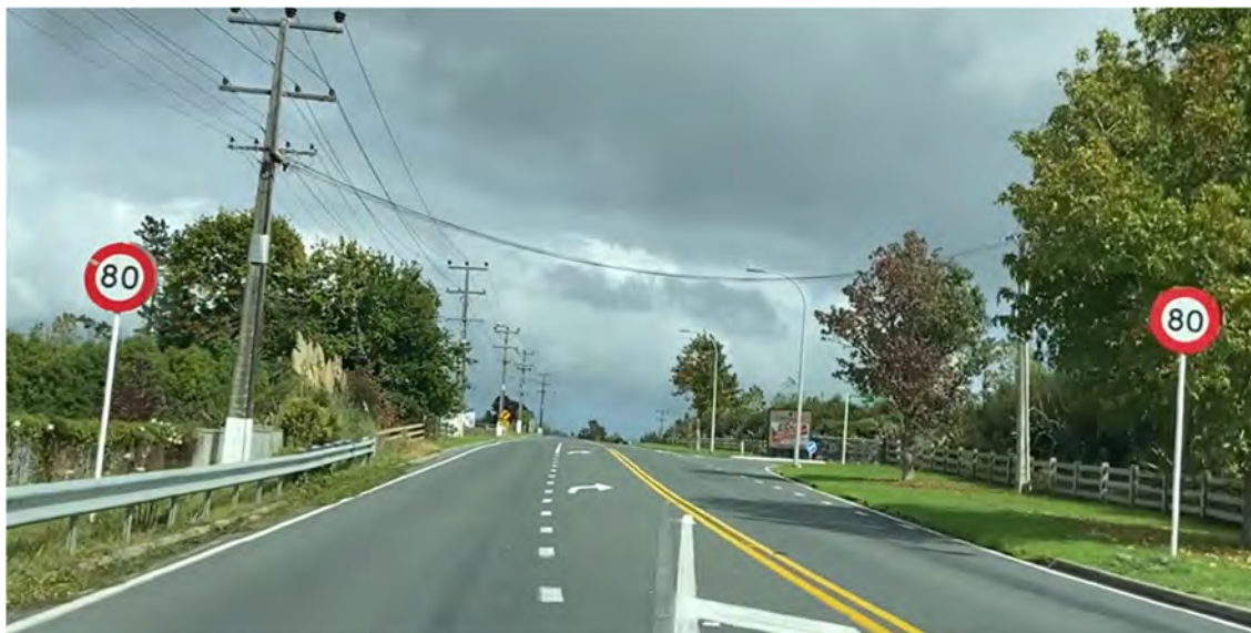
Figure 2-5: Existing SH16 configuration along site boundary travelling westbound approaching MacLennan Farm Lane (shown on left hand side)
