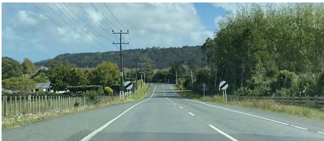
Figure 2-6: Existing SH16 configuration along site boundary travelling westbound after MacLennan Farm Lane
