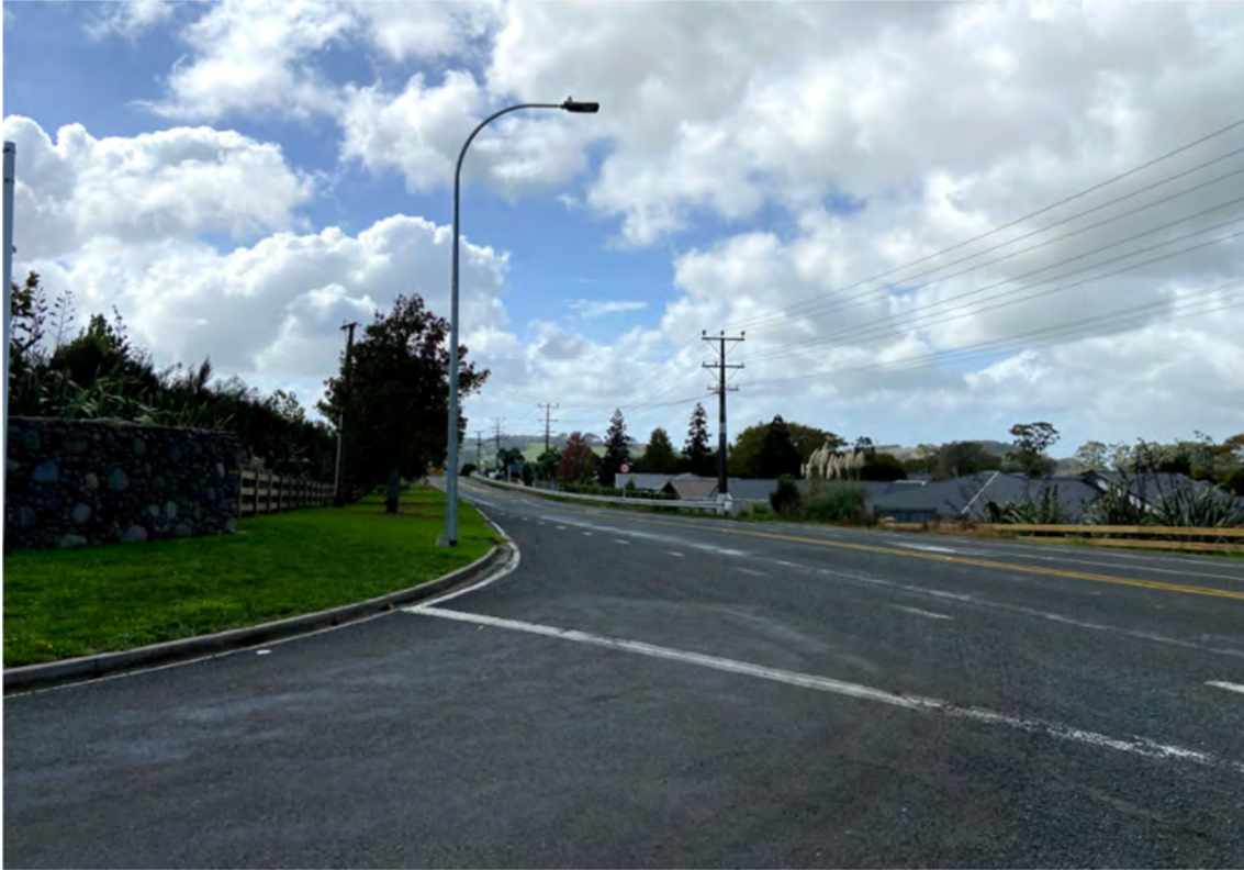
Figure 2-7: SH16 / MacLennan Farm Lane Intersection Looking East
