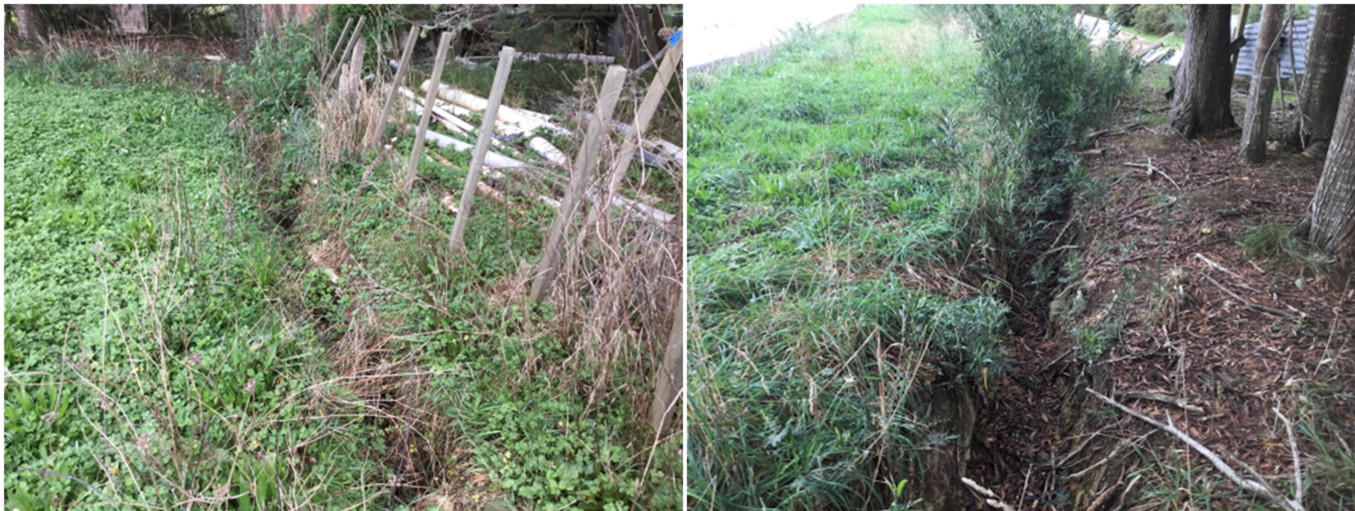
Plate 5 & 6. The drain linking the northern wetland with the unnamed tributary of the Rangitopuni Stream. It is linear, has a narrow, excavated channel and does not meet the criteria as a stream; however, we understand that the AUP considers this to be a stream (shown as a continuation of Stream I1 on Figures 4 and 5).
