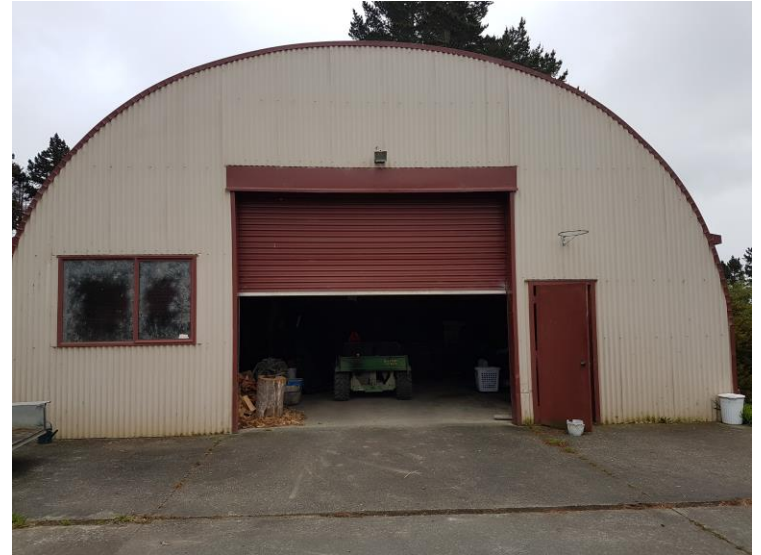
Painted Tin Barn
