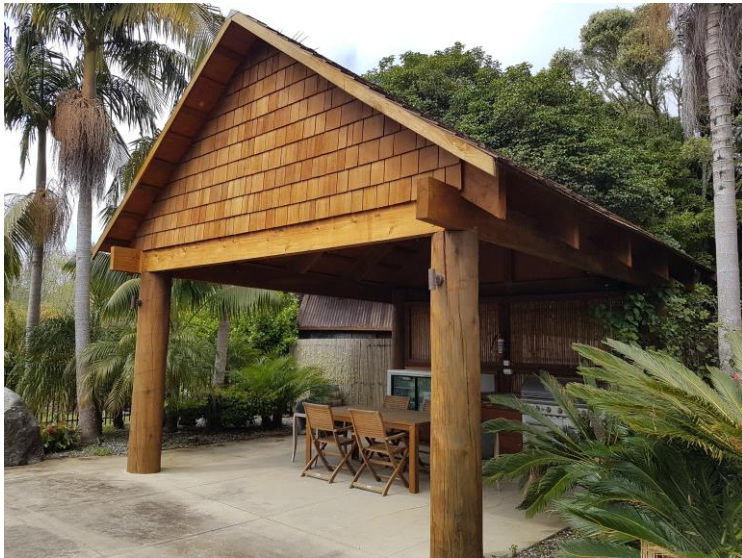
Unpainted Wooden Pergola with Tiled Roof
