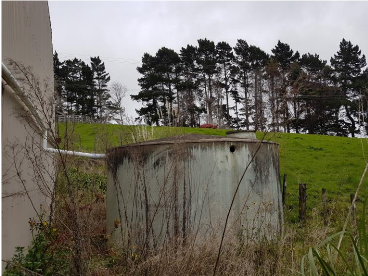
Concrete Rain Water Tank
