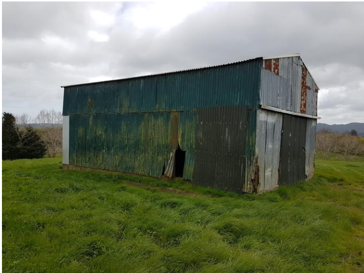
Painted Tin Shed
