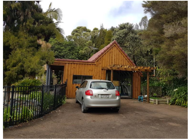
Unpainted Wooden Residential Unit
