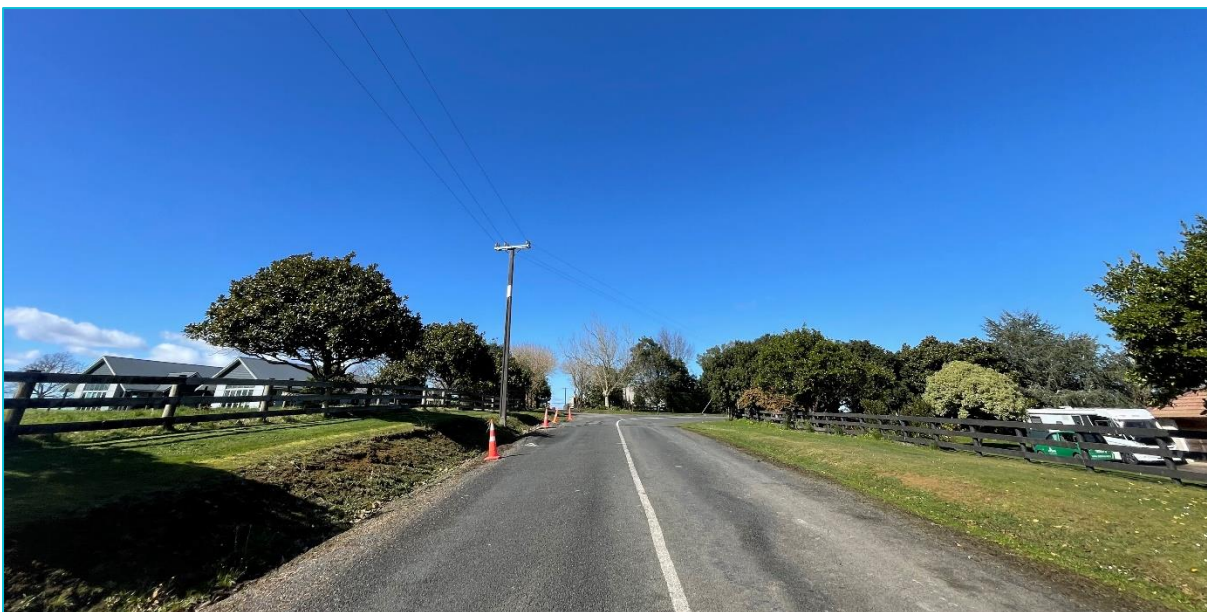
Figure 4-17: Sim Road looking east near the location where the new road deviates away from the existing alignment. Photo taken from outside proximate 77 Sim Road. (Source: MJ_IJL)
