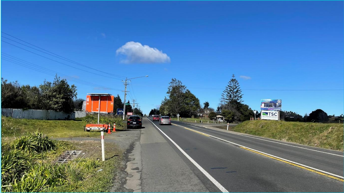
Figure 4-30: Looking south from Paerata Road (SH22) at the intersection with Butcher Road. The proposed alignment connects NoR 7 from the west (right) across to NoR 4 to the east (left). (Source: MJ_IGL)
