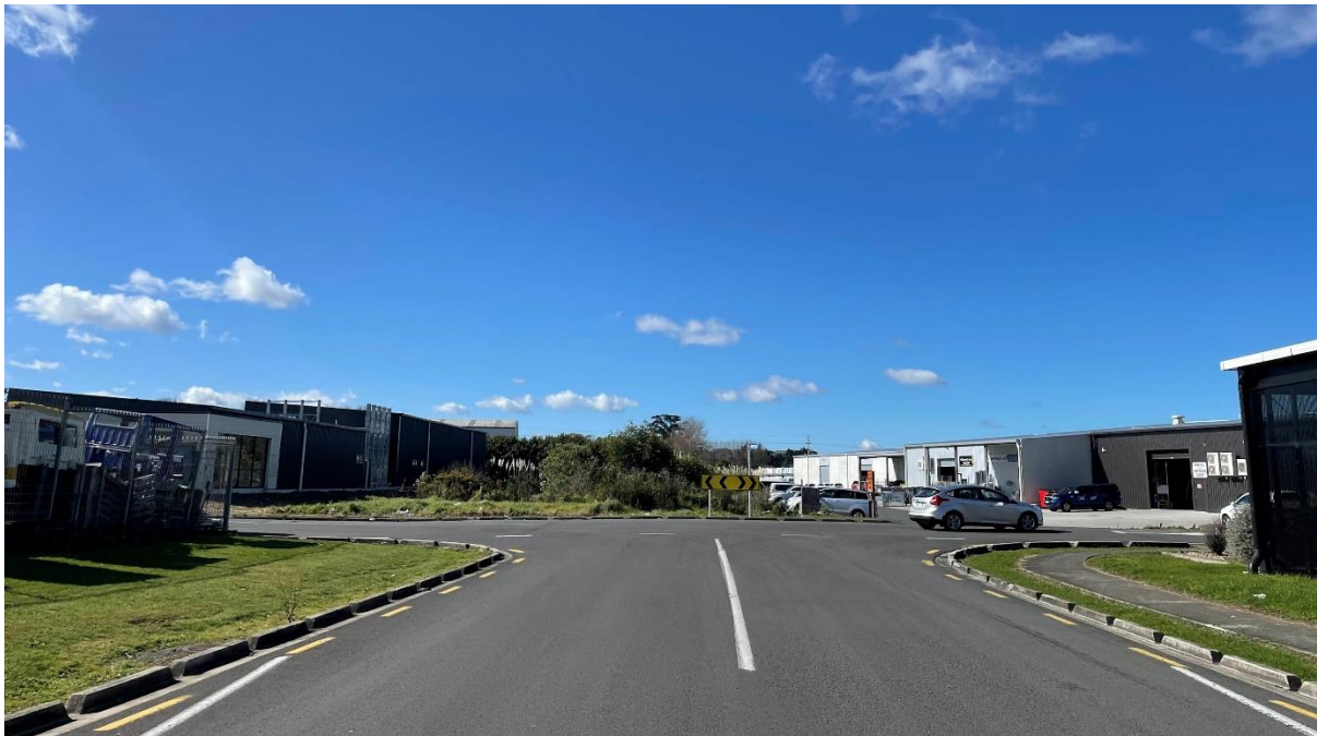
Figure 4-36: Looking east from Svendsen Road (near the intersection with Crosbie Road) toward the vegetated culvert which extends toward the NIMT. (Source: MJ_IGL).
